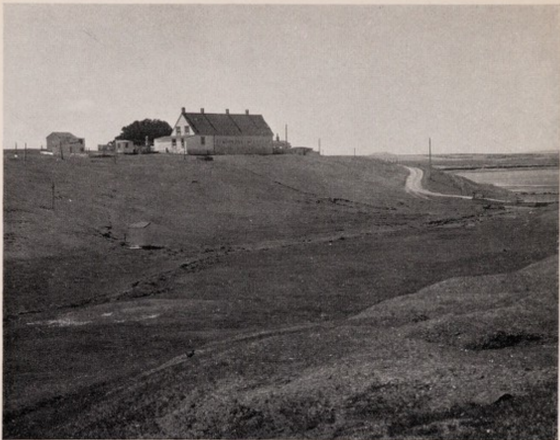
The house at Port Louis which incorporates the old English fort (which was the original Government House until the removal of the capital to Stanley in 1844).
