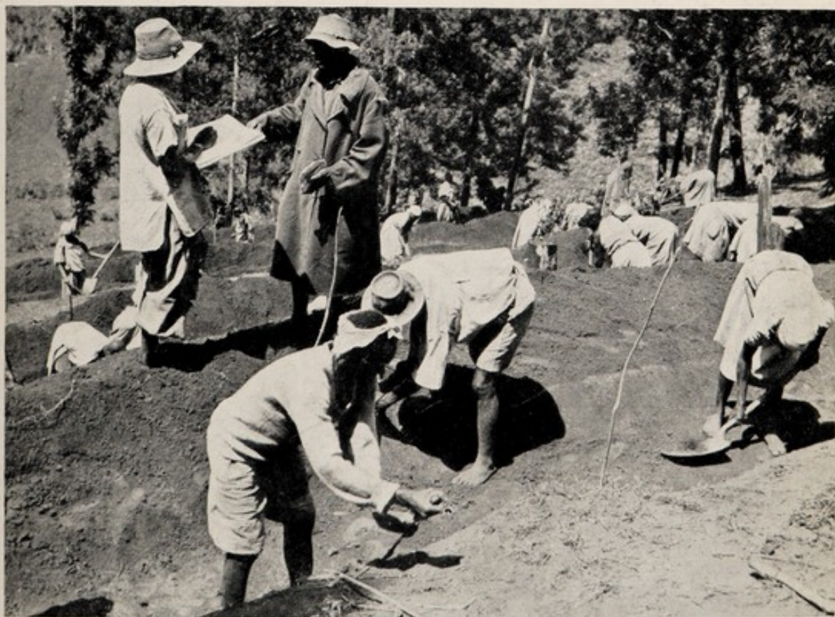
THE BATTLE TO SAVE THE SOIL: CONTOUR TERRACING IN PROGRESS
