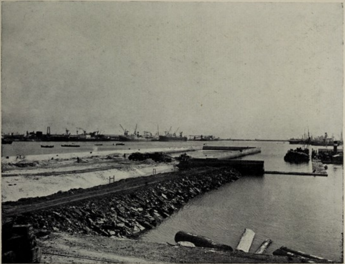
CONSTRUCTING THE NEW TIMBER WHARF AT TAKORADI HARBOUR
