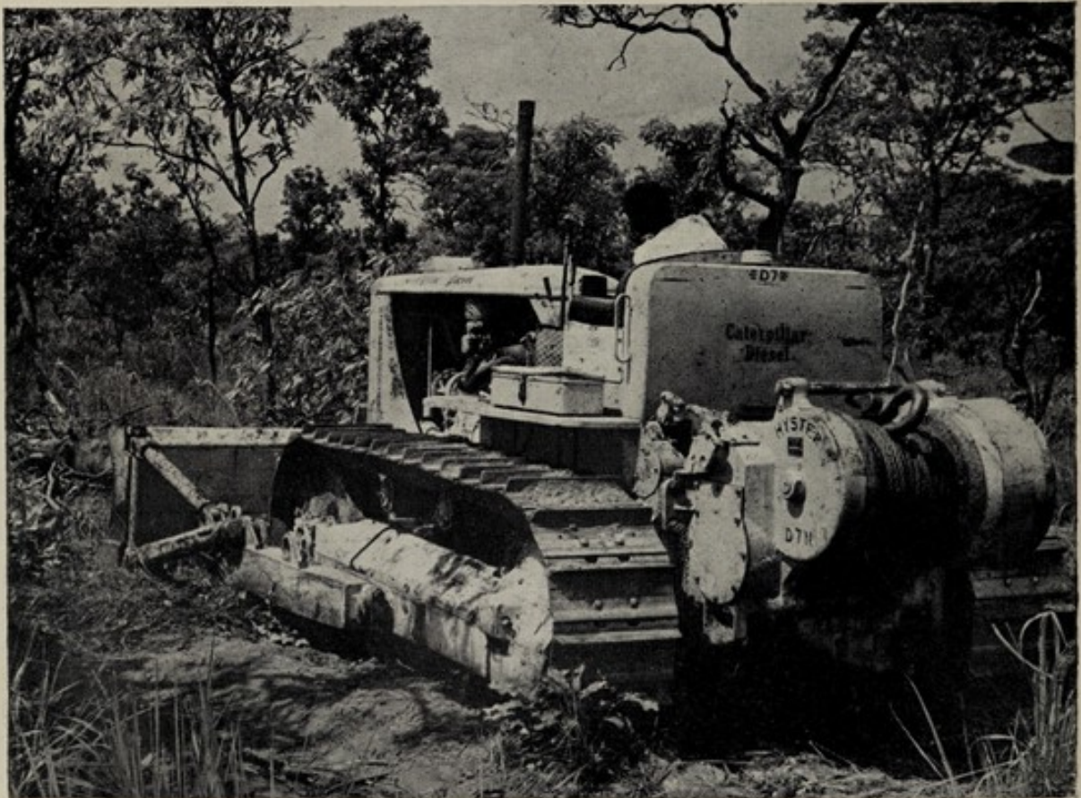
CLEARING THE BUSH AT DAMONGO
