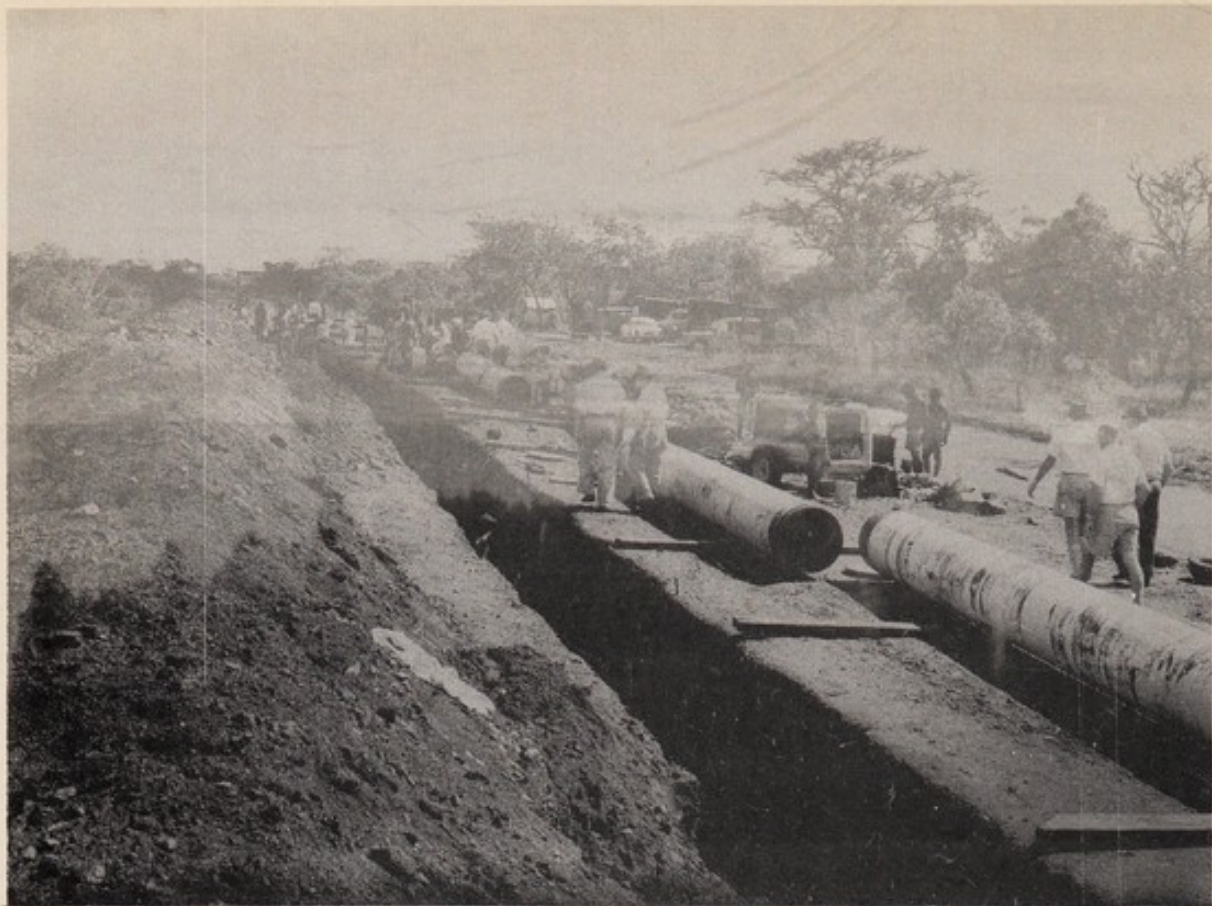
Laying the Walker Ferry pipeline, which will eventually stretch 29 miles and rise 2,500 feet, supplying Blantyre/Limbe.
