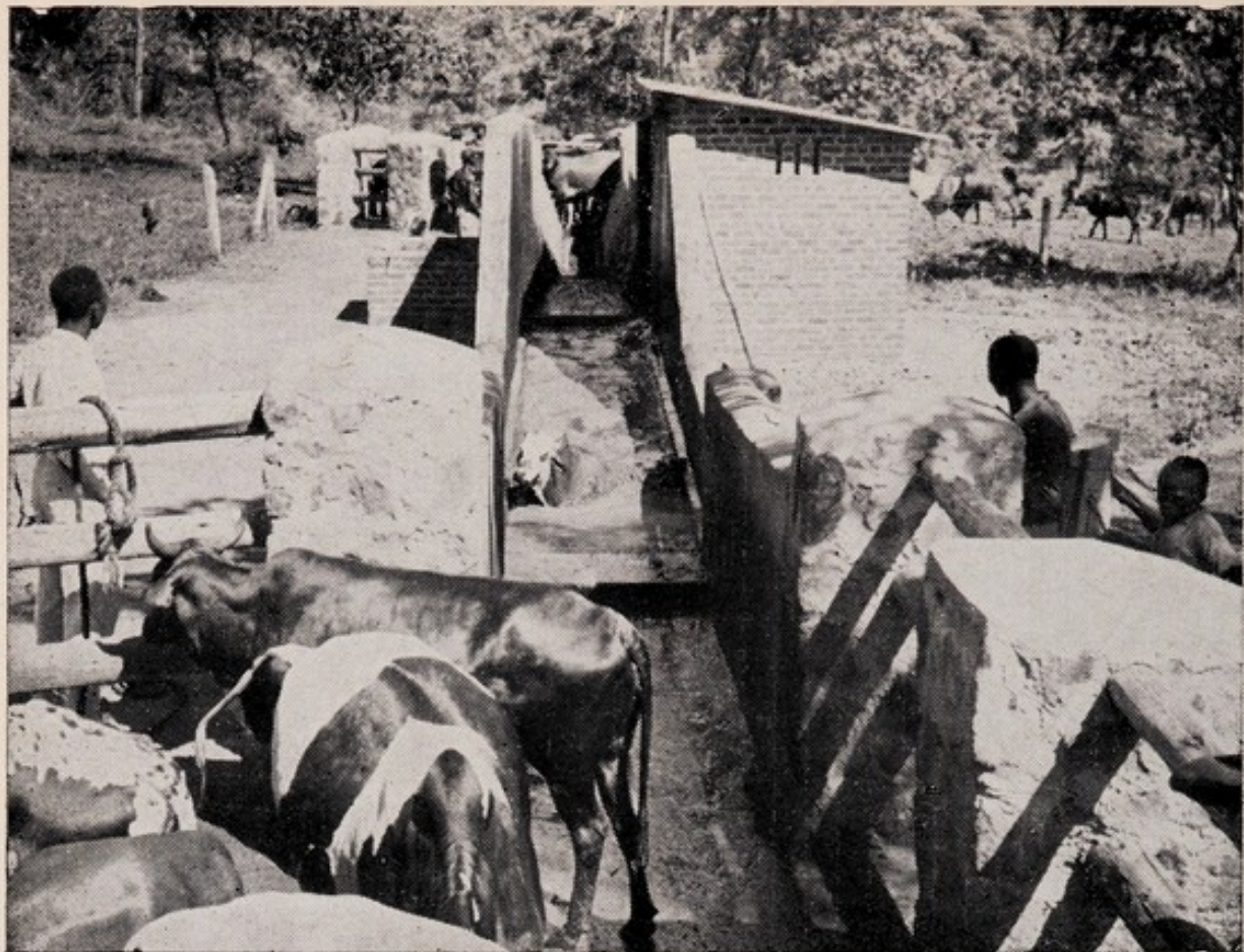
Under a Colonial Development and Welfare Fund scheme, money has been provided for the extension of dipping services throughout Nyasaland. This prefabricated steel dipping tank has been so designed that it can be assembled on site and installed.
