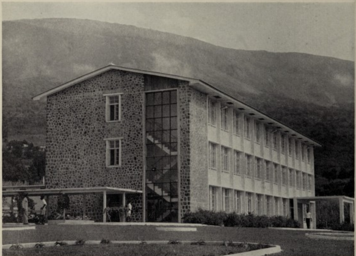
New Ministerial Building, Buea
