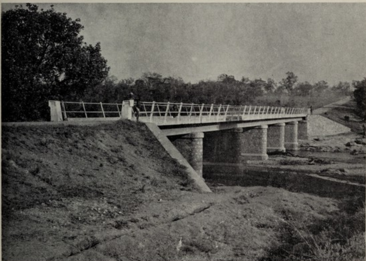
New bridge construction, Berli-Serti Road, 1957.
