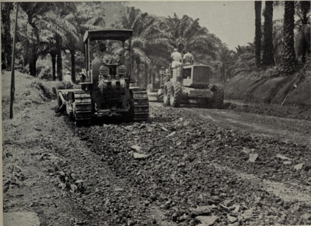
Construction work on the VICTORIA TIKO Road—scarifying old road surface.
