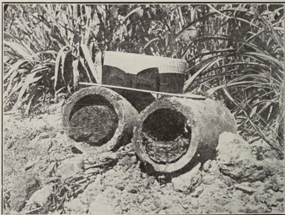
Evils of a defective siphon illustrated. The sludge has escaped into the sub-surface tiles which have been uncovered.
