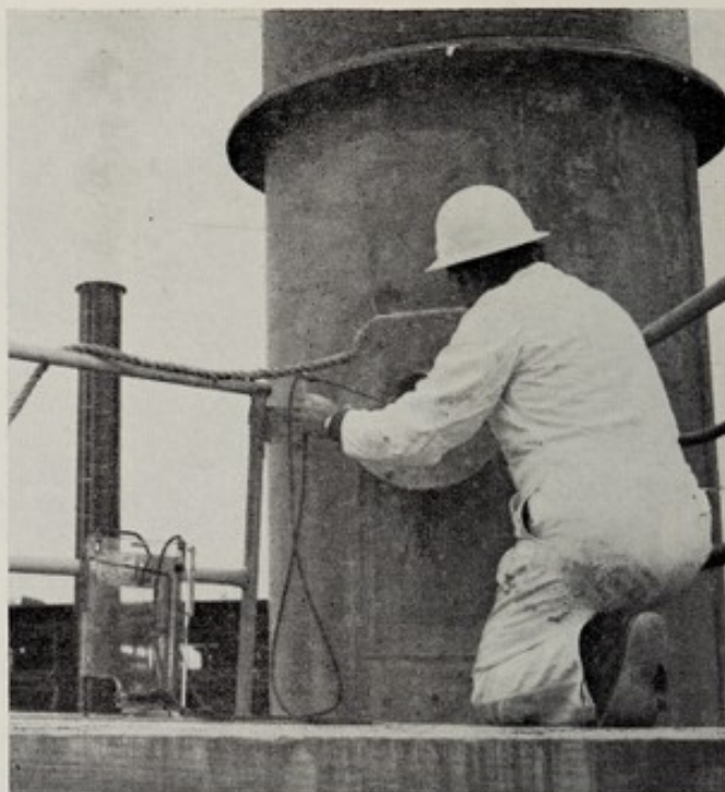
16. Air Pollution—Industrial sources of pollution, such as chemical works, are required to control emissions which are tested regularly by departmental inspectors. This test is being made by Mr Ek Tieng Lee, a Colombo Plan engineer from Singapore.
