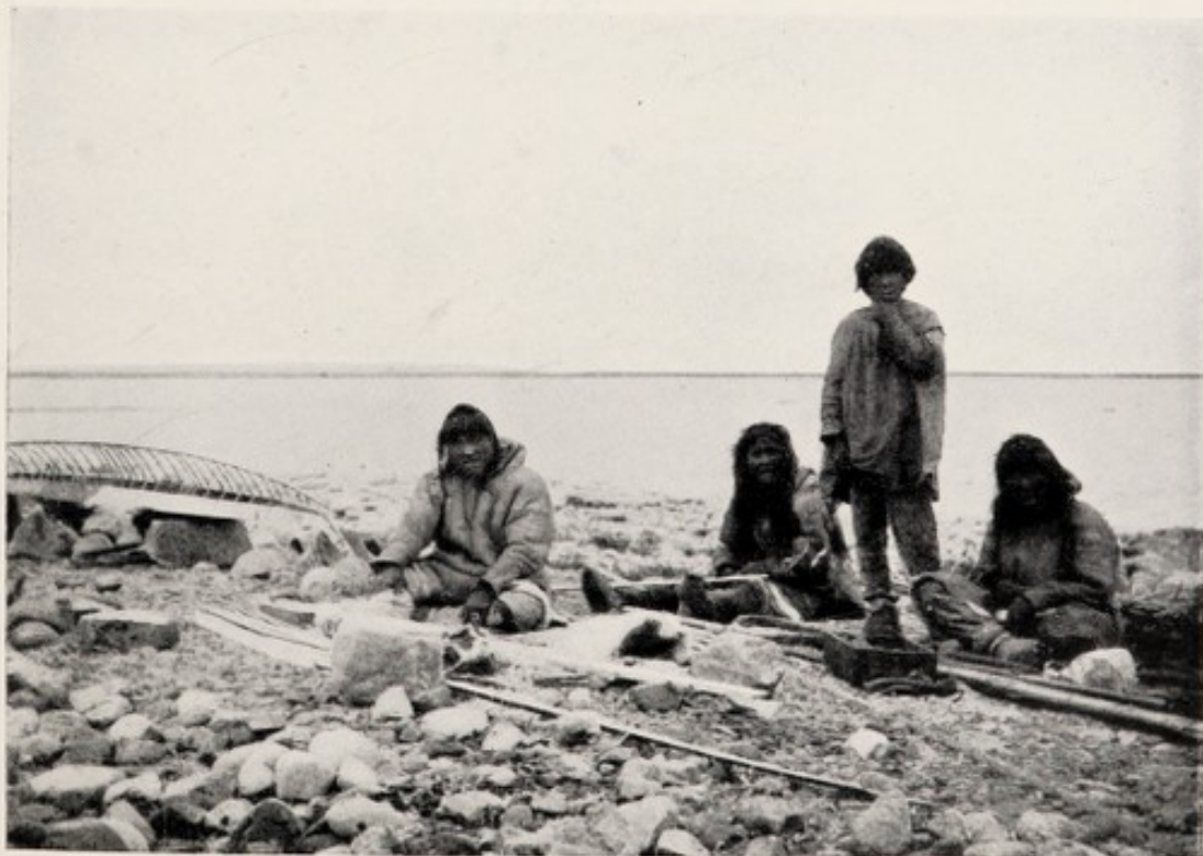
BUILDING KYAKS, HUDSON BAY.
