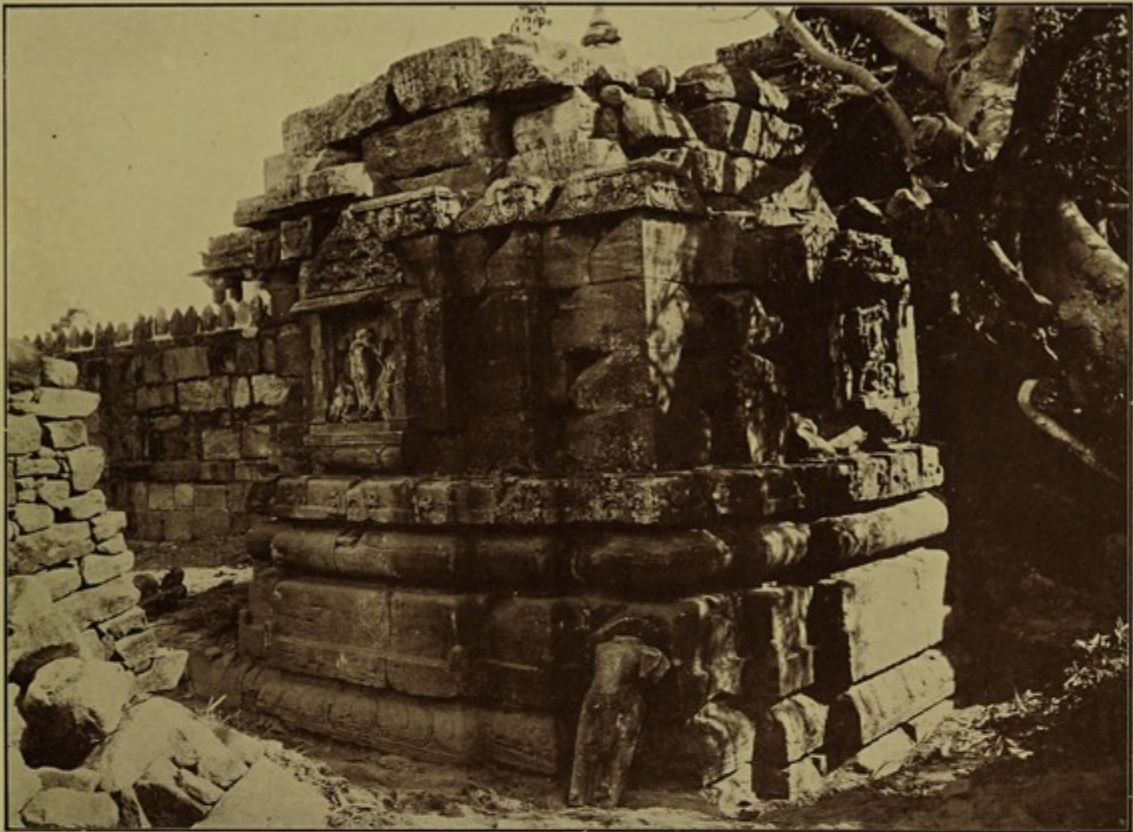
OLD SHRINE BESIDE THE TEMPLE OF SURYA AT THAN, FROM THE NORTH-WEST.
