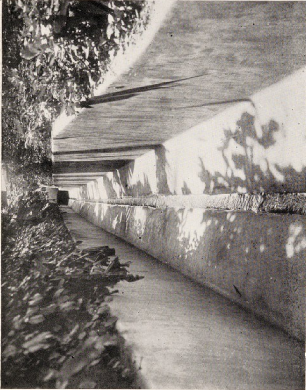
FIG. 4.—A LARGE CONCRETE DRAIN TO CARRY OFF STORM WATER, TRINIDAD.
