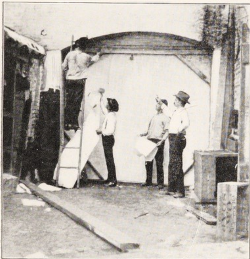
FIG. 26.—PAPER-SCREENING AN ARCHWAY PREVIOUS TO FUMIGATION, NEW ORLEANS. p. 140]
