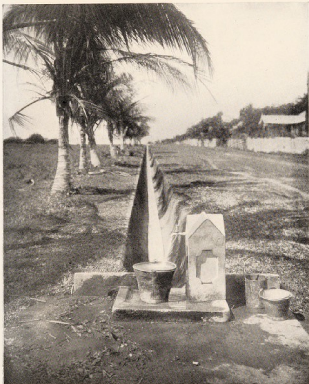
FIG. 2.—A WELL-CONSTRUCTED DRAIN AND STANDPIPE, THE AGENTS WHICH HAVE CAUSED THE DIMINUTION OF MOSQUITOS, TRINIDAD. p. 12]
