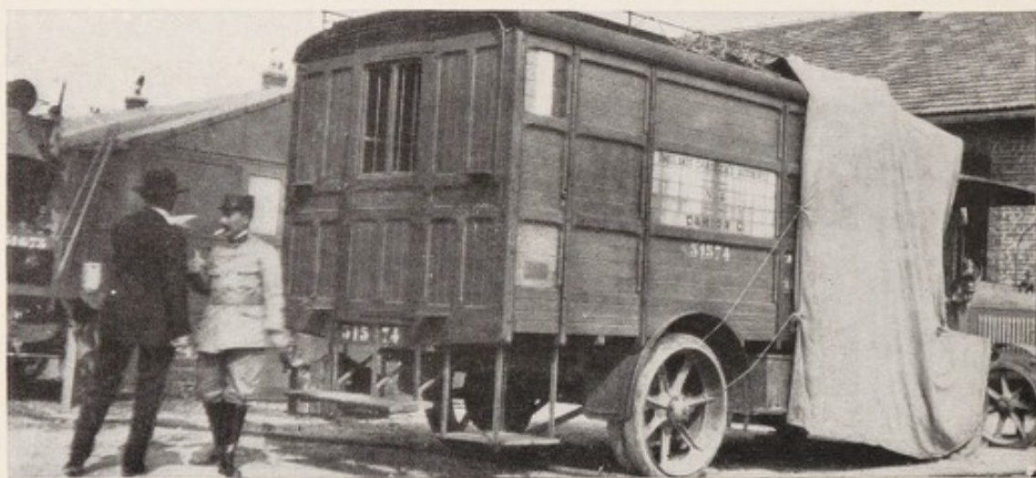
Fig. 86.—Showing truck No. 3 which contains the electric-light motor at the forward end and storage space at the rear for operating-room linen. (See page 62.)
