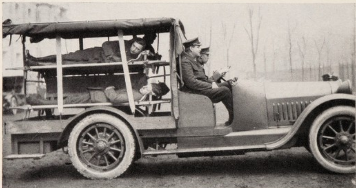
Fig. 102.—Type of heavy motor ambulance used at the American hospital and designed to carry four patients. (See page 68.)
