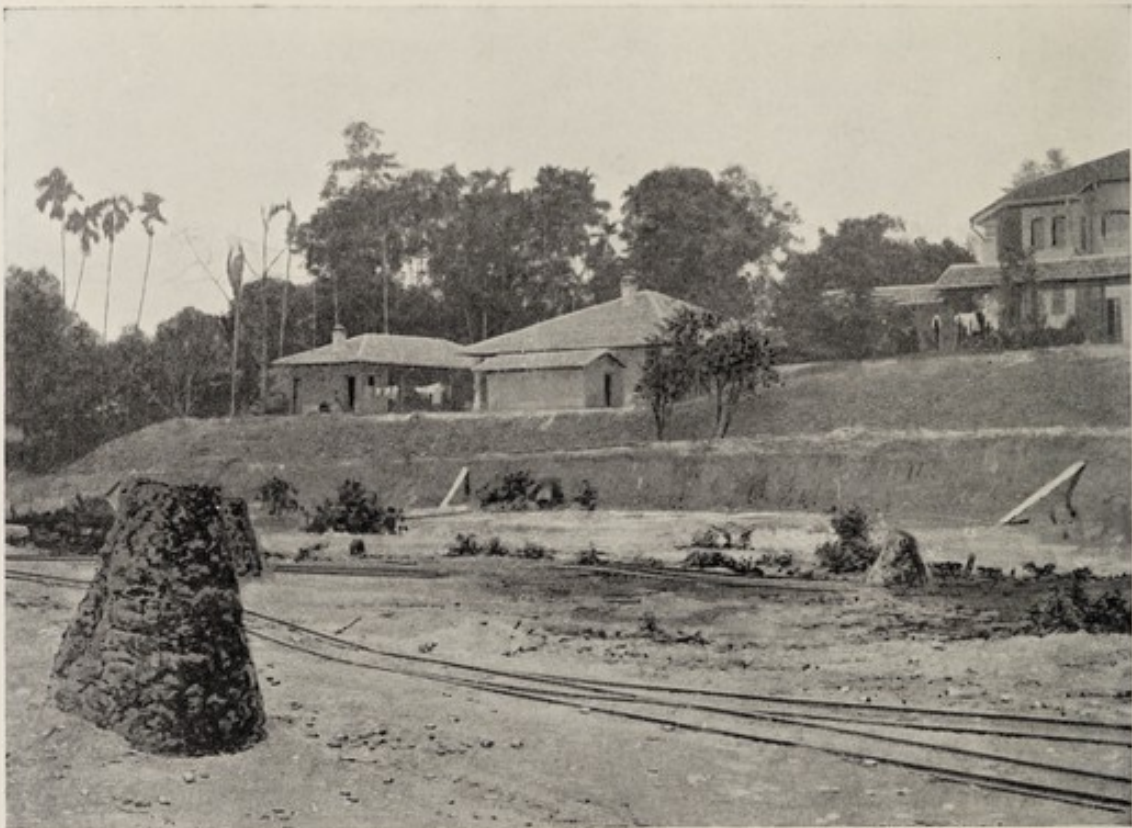
Shows the situation of some of the houses on the hill in relation to the proposed filter beds in the valley.
