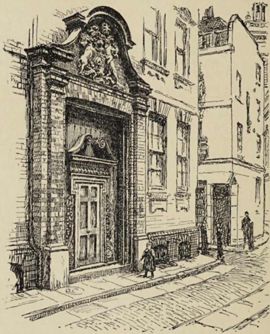
INNOLDERS' HALL. ENTRANCE DOOR
