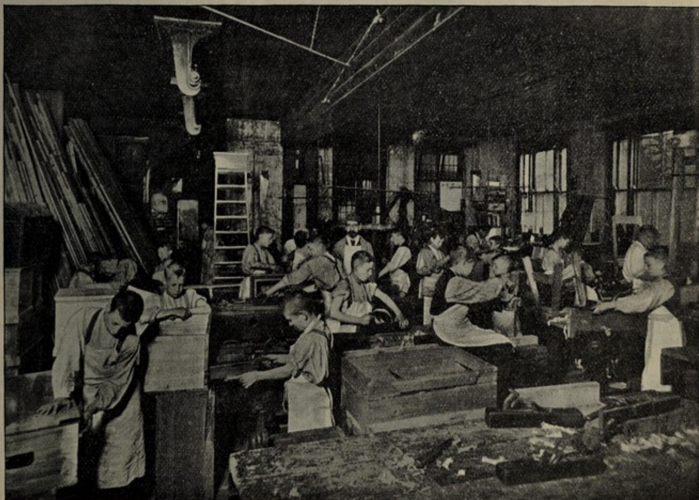
CARPENTERS AT WORK AT STEPNEY CAUSEWAY, LONDON, E.
