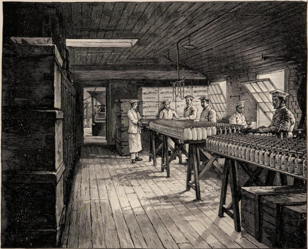
STEAM DRYING CUPBOARDS AND WRAPPING ROOM.
