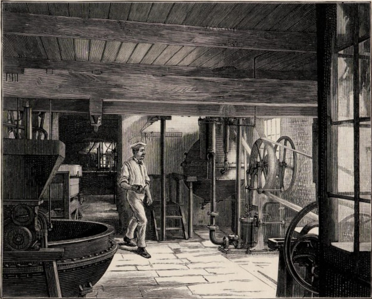
TRANSFORMER AND VACUUM PAN.
