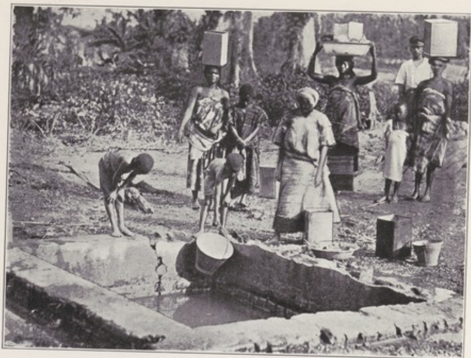
Another important water supply of Kumasi in 1924. Note Use of many dippers, broken coping, cracked wall and surrounding puddles.
