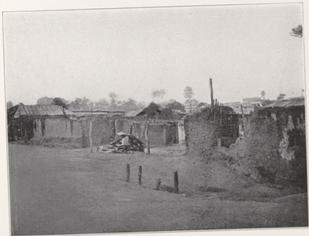
After the thatched roofs had been burnt by their occupants the buildings were demolished in many cases as the rooms were often only 6 ft. by 4 ft. by 5 ft. in size and were unprovided with either lighting or ventilation.
