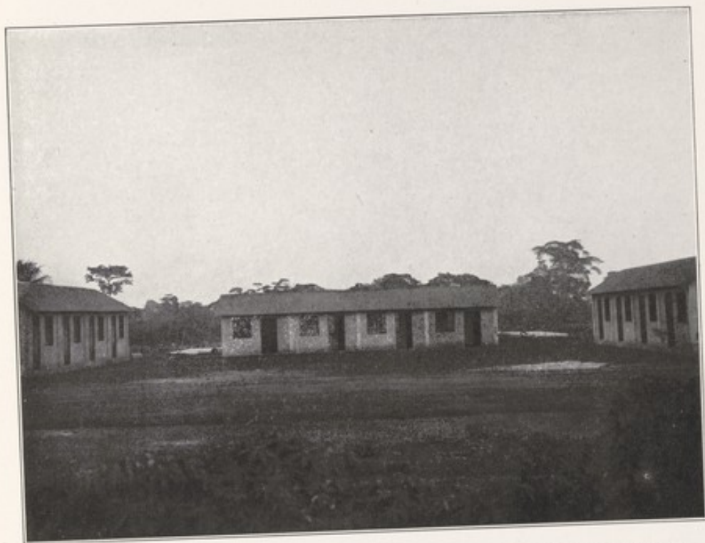
Part of the New Zongo Housing Scheme. (Buildings not yet completed and construction of sanitary structures not yet commenced.)
