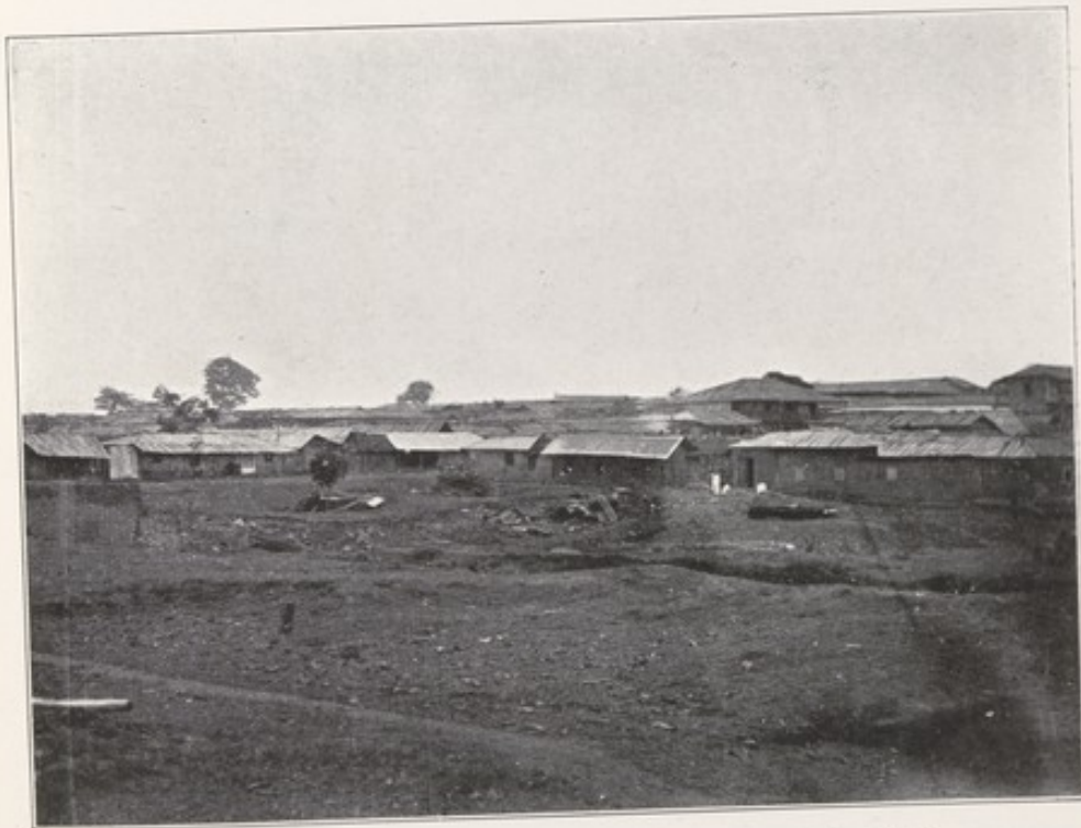
The badly infected portion referred to above after demolition. The inhabitants were evacuated to a temporary camp.
