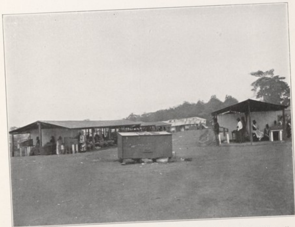
New sheds erected in the Zongo Market, Kumasi to replace the insanitary "Buggas" demolished in June. Note Butchers stalls with flyproof safes, washable cement tables and floor. Flyproof Dustbin in foreground.
