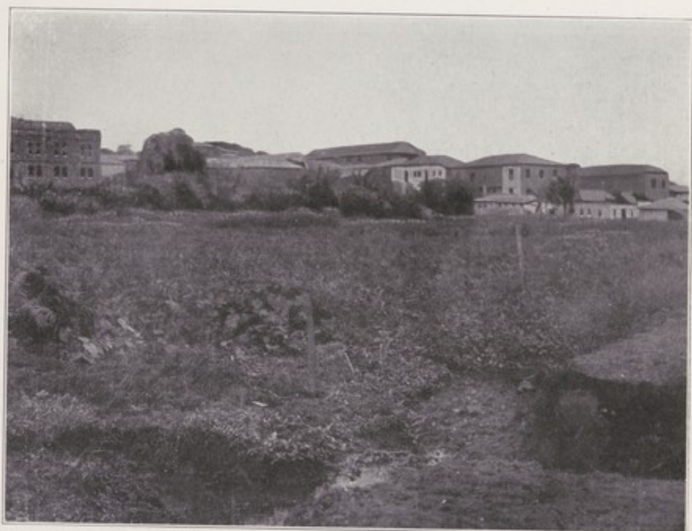
Another swamp at present being filled-in.
