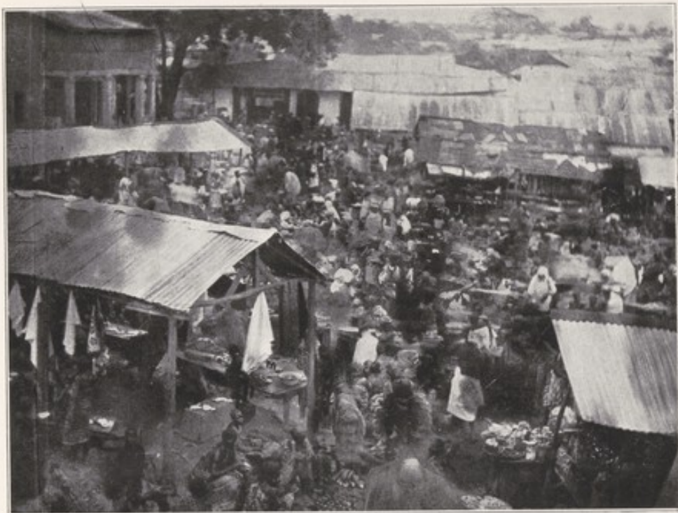
Kumasi Market. Congested and difficult to cleanse.
