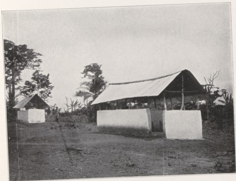
Modified Salga-type latrine constructed at Bantama, Kumasi, in July, 1924.
