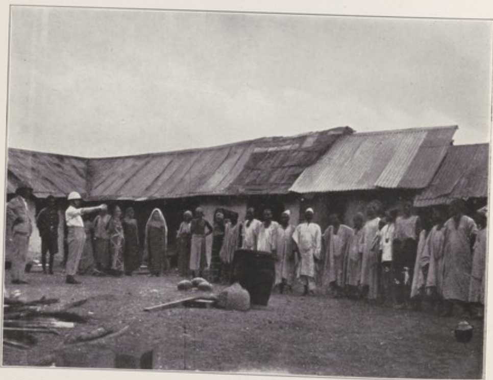
The above after removal of hovels. A few the occupants of the compound can be seen.
