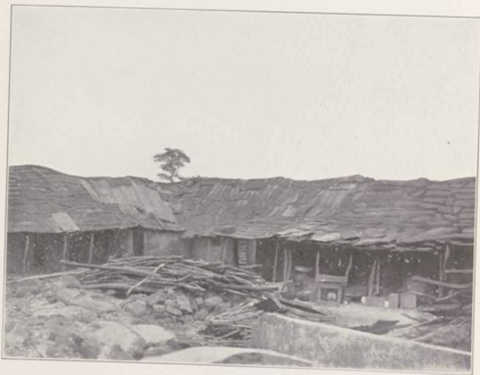
Another type of insanitary house in which several cases of Plague occurred. The heap of swish and sticks in the foreground resulted from the demolition of a number of hovels covering the Compound itself.
