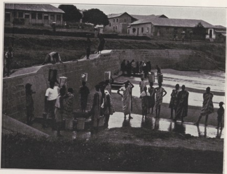
The Odum Wells — The chief water supply of the Native population. The well in the foreground is reserved for Europeans. Many dippers are used and the water is liable to fouling.
