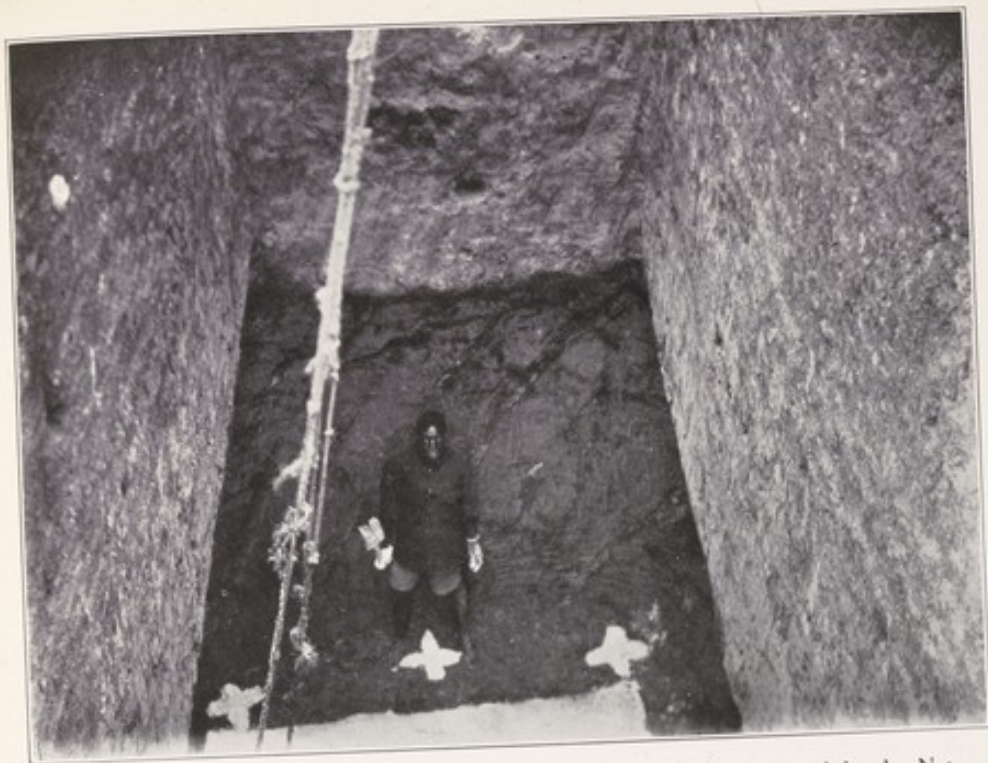
To show depth to which latrine pits are dug—26-30 feet below ground level. Note under cutting of deeper portion of pit to increase capacity.
