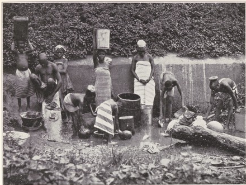
An important water supply of Kumasi in June, 1924.
