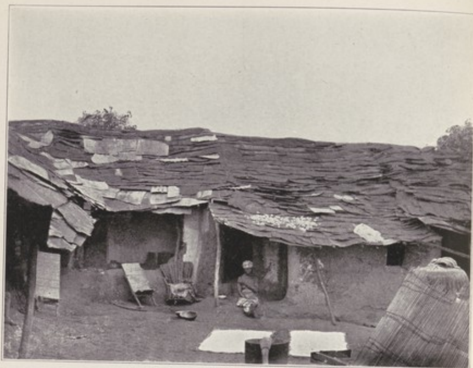
A. type of Plague infected compound which was later demolished. Note the verandas and annexes which prevented light and air reaching the living rooms.
