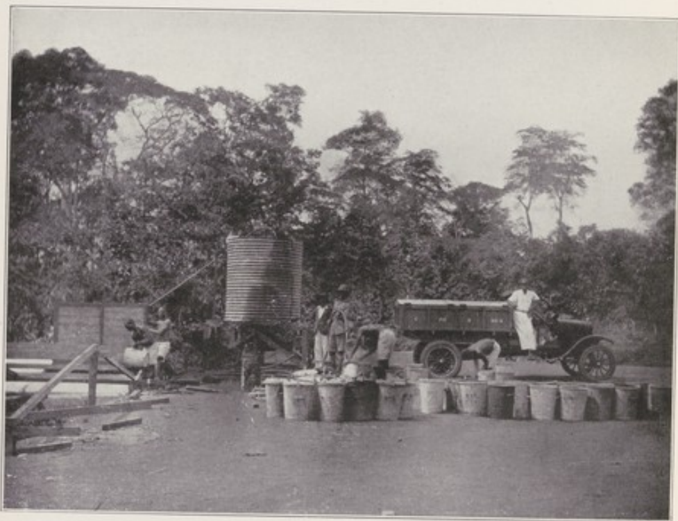
Night-Soil Depot. Motor conservancy system replacing carriage of night-soil through streets by head load.
