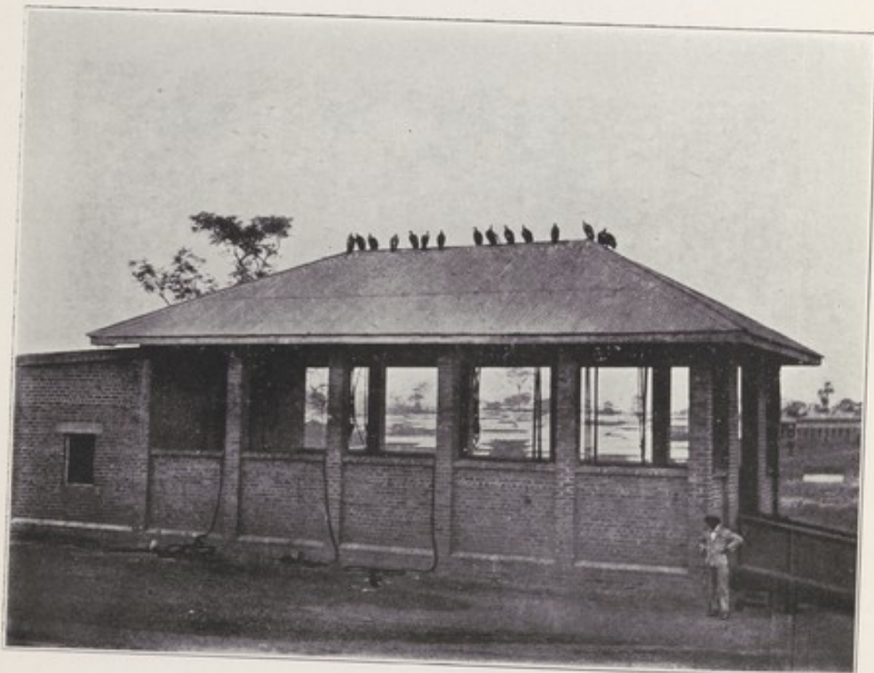
Kumasi Slaughter House. The building is inadequate in size and no means exist of flushing it with water. On the roof are a number of vultures. The presence of this bird is a reflection on Kumasi. The assistance of such foul feeders in dealing with town refuse should not be required.
