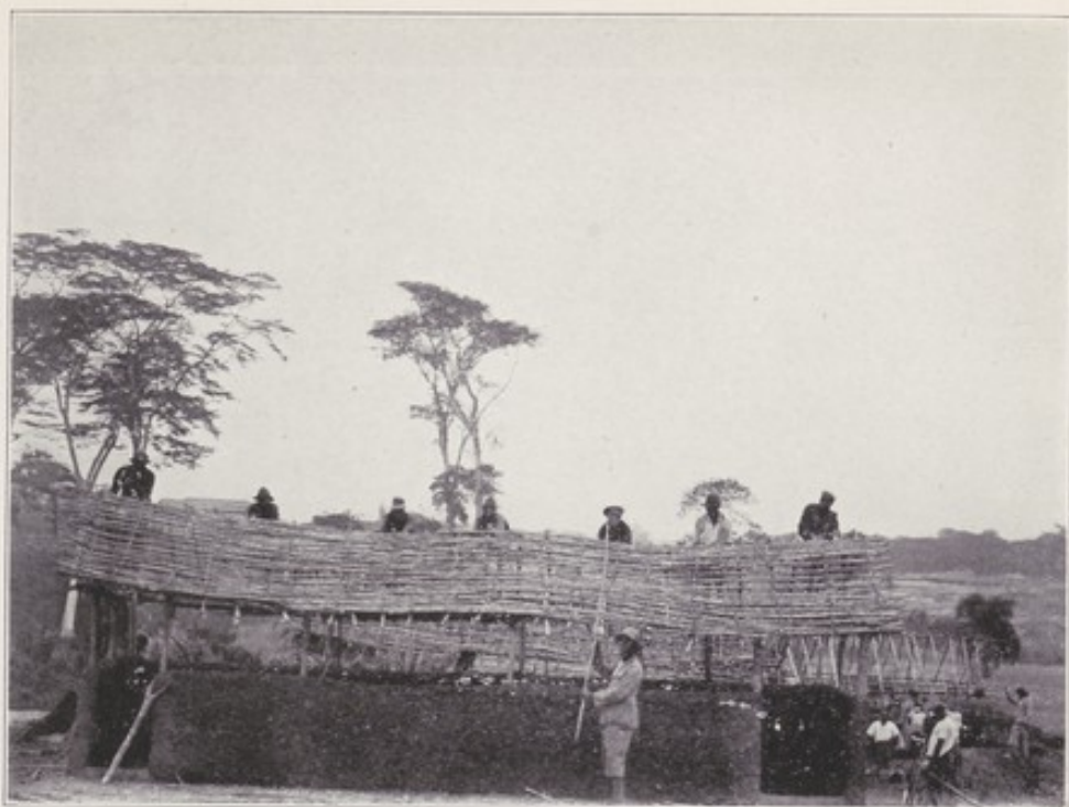
Roofing a modified Salga-type latrine.
