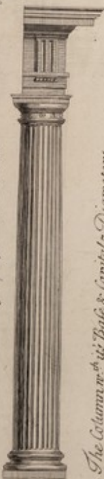
The Column with its Base & Capital 8 Diameters
