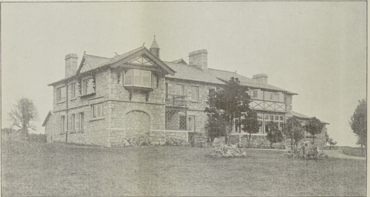
WESTMORLAND CONSUMPTION SANATORIUM.—VIEWED FROM THE SOUTH-WEST.
