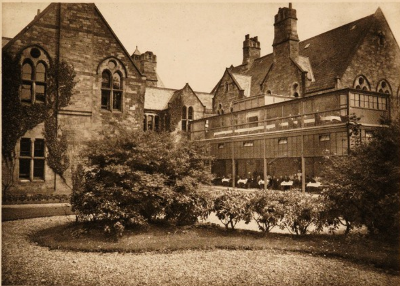
ASHTON WING: NEW VERANDAHS
