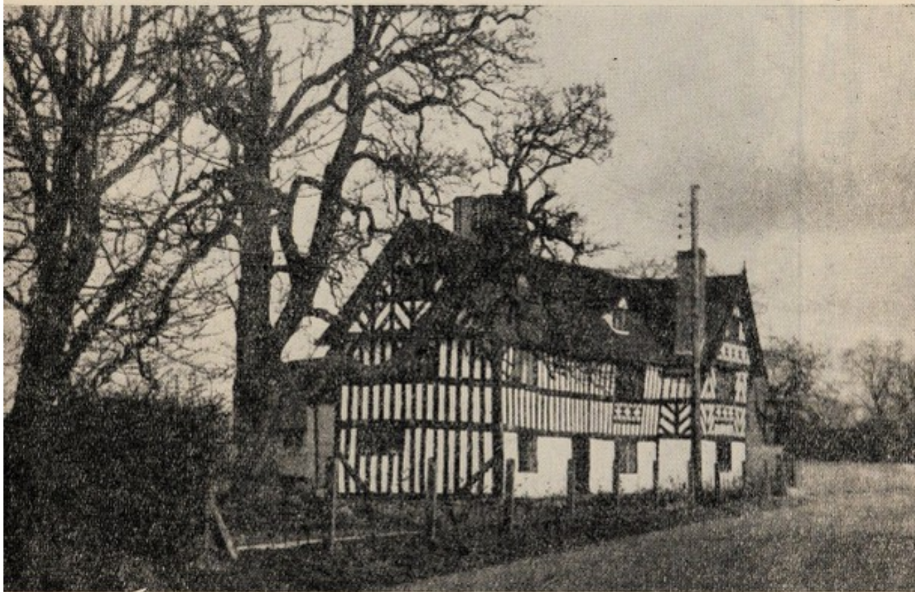
Examples of Dwellings of an age and type difficult to make completely fit but which should be preserved for their architectural merit—a "cruck" cottage (top) at Haughton and Haughton Old Hall.
