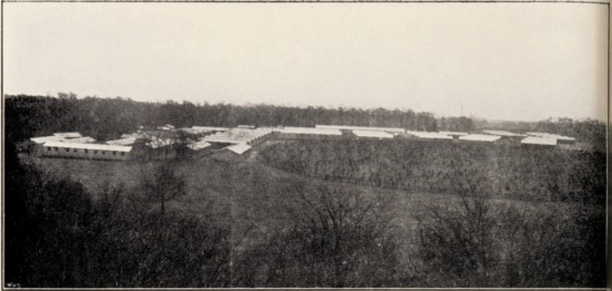
General view of Hutment
