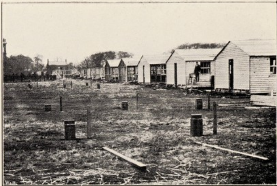
General view of Hutment.
