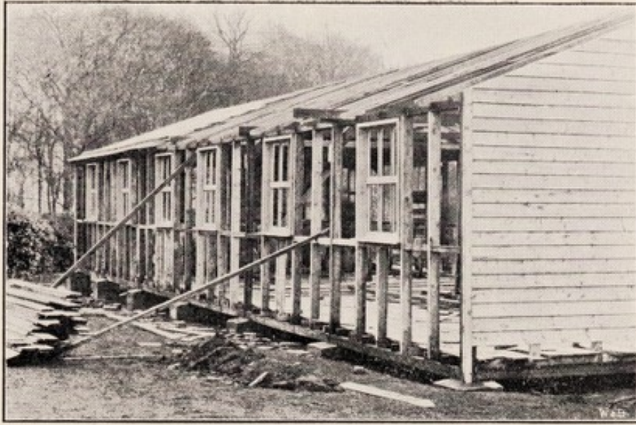
Framework of hut.
