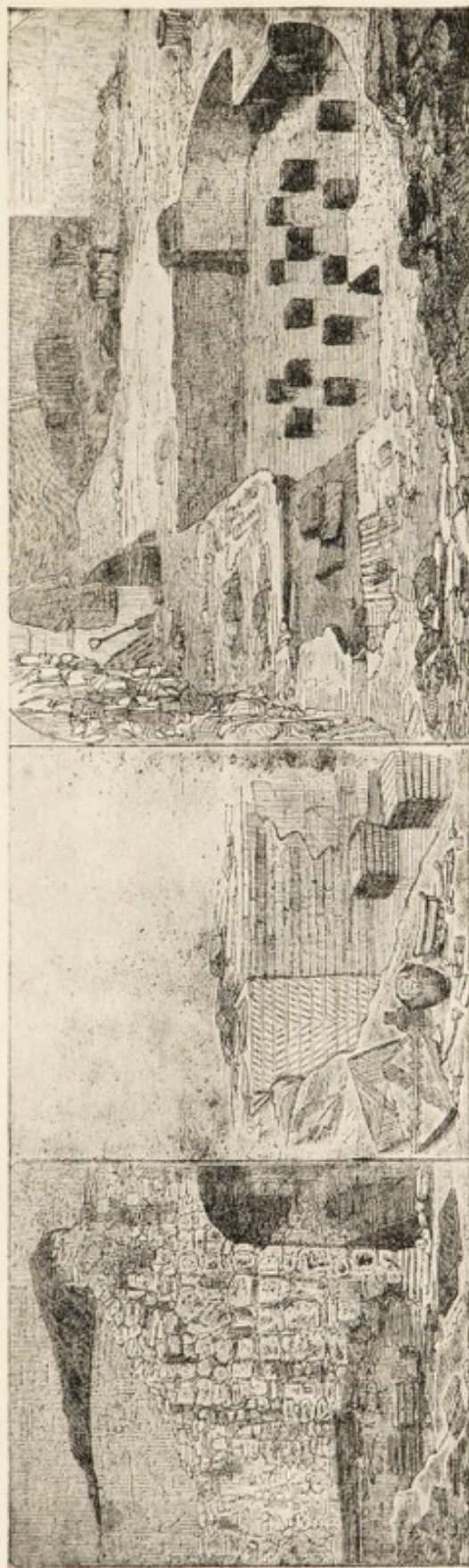
A. B. C. FIG. 25.—(A, old masonry; B, brickwork with a flue tile; C, foundations of chamber.) Foundations discovered in Lower Thames Street in 1859.
