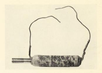
Helix of copper wire and bar magnet used by Faraday. It was with this apparatus that he first induced an electric current by plunging the magnet into the coil
