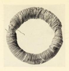
Historic ring of soft iron, wound with separate coils of copper wire connected to battery and galvanometer respectively, used by Faraday in his first successful experiment in electro-magnetic induction
