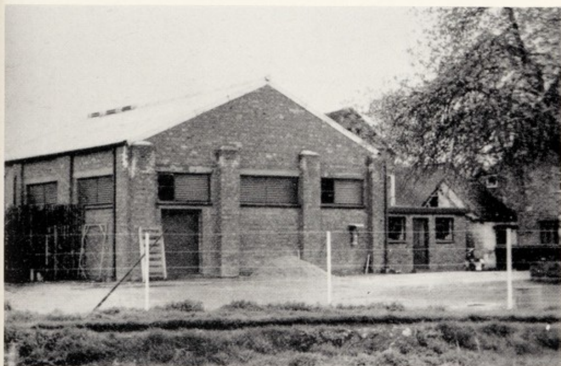
EASTWYKE FARM SLAUGHTER HOUSE (REMODELLED 1963)
