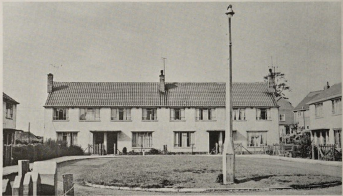
NEW HOMES FOR OLD. The building of houses is an essential part of the Slum Clearance Programme.
