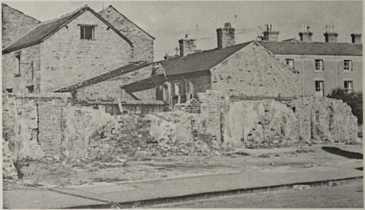
GONE! Site of 28—46 Roft Street after demolition.
