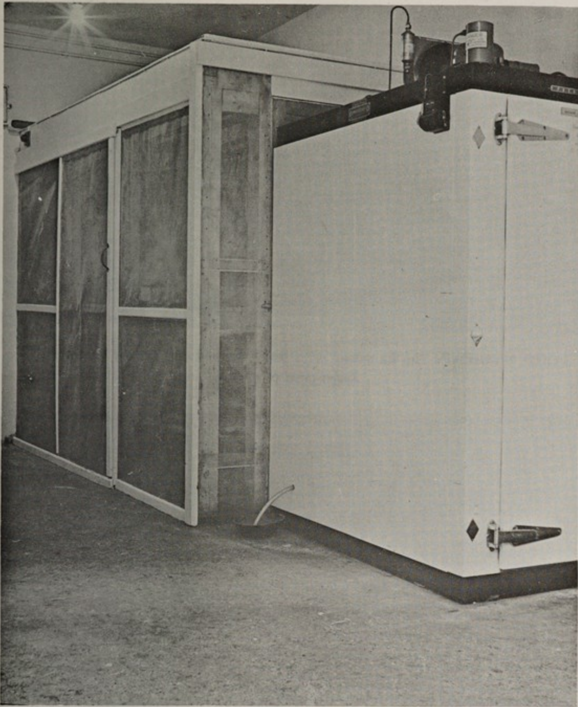
FOOD HYGIENE. Zinc-meshed Bacon Store and Refrigerator for cooked meat storage, provided by grocer at the request of the Public Health Inspector.
