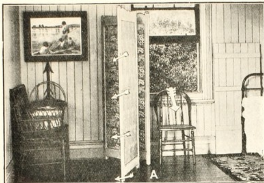
(A) Good ventilation. Lower sash raised, no oblique wind. White arrows show cool, pure, "white" air; black arrow shows used-up, poisoned, "black" breath—not air. (Details on opposite page.)
