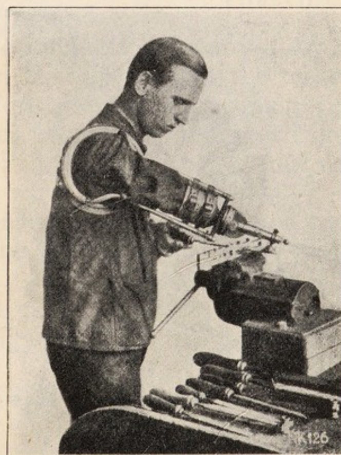
FIG. 141.—Shortened ball connection, with rubber presser.
