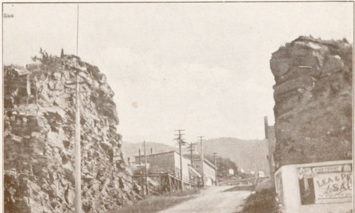
View of street cut through solid rock in a city in Western Canada. To utilize the lots facing this street the rock has to be removed from the building sites at great expense.
