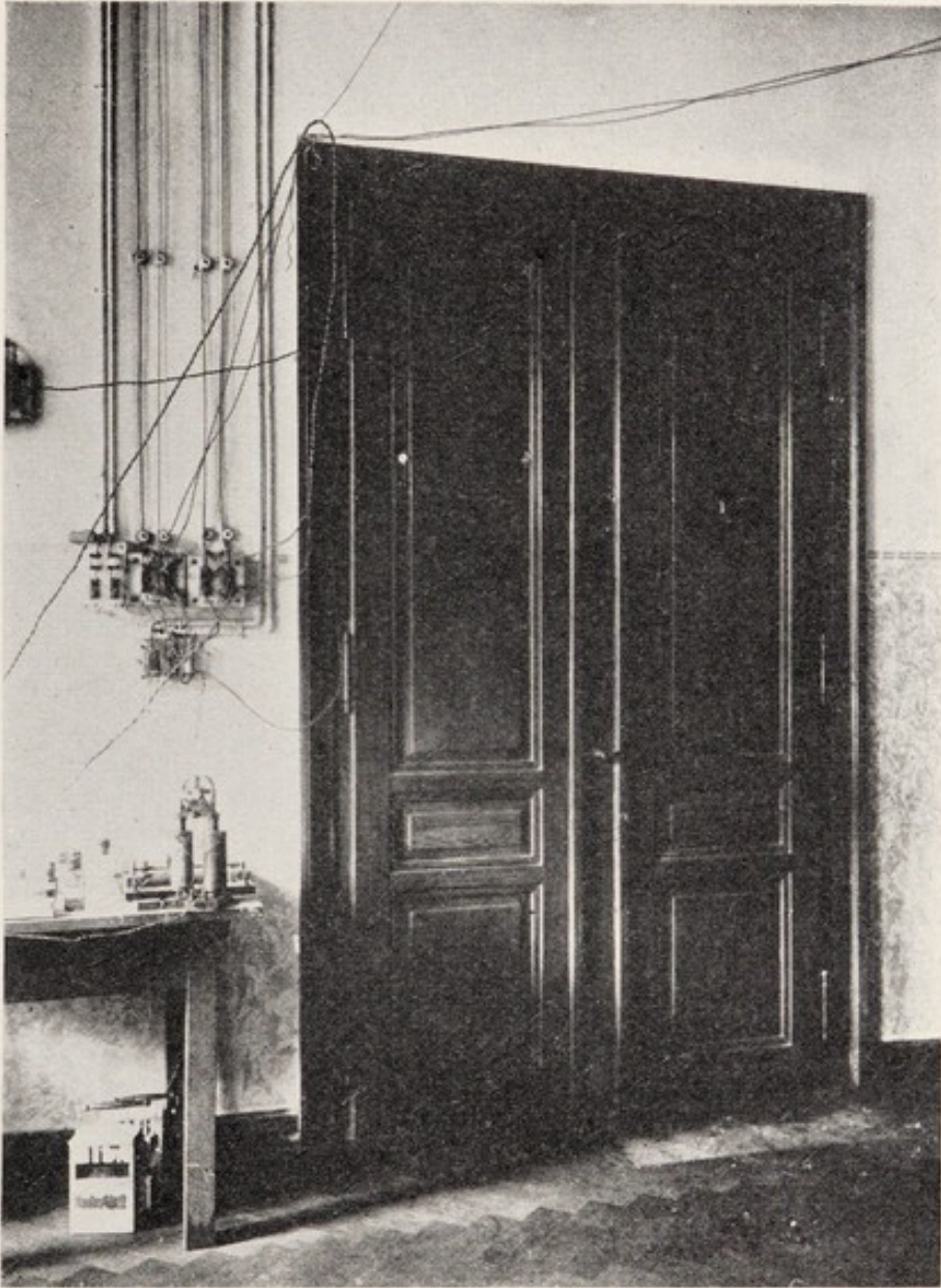
FIG. 20. The famous door which Roentgen is said to have dismantled to determine why X-ray photographs taken through it showed streaks and bands of decreased density. He demonstrated that the marks were shadows cast by white lead used in cementing the panel mouldings.
