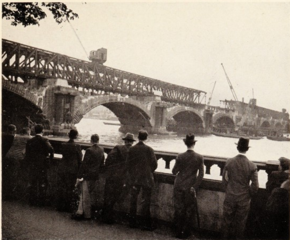
86 The Demolition of Waterloo Bridge, 1938
