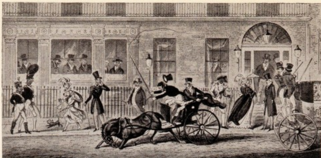
54 "Exterior of Fishmongers' Hall: a Regular Breakdown"
