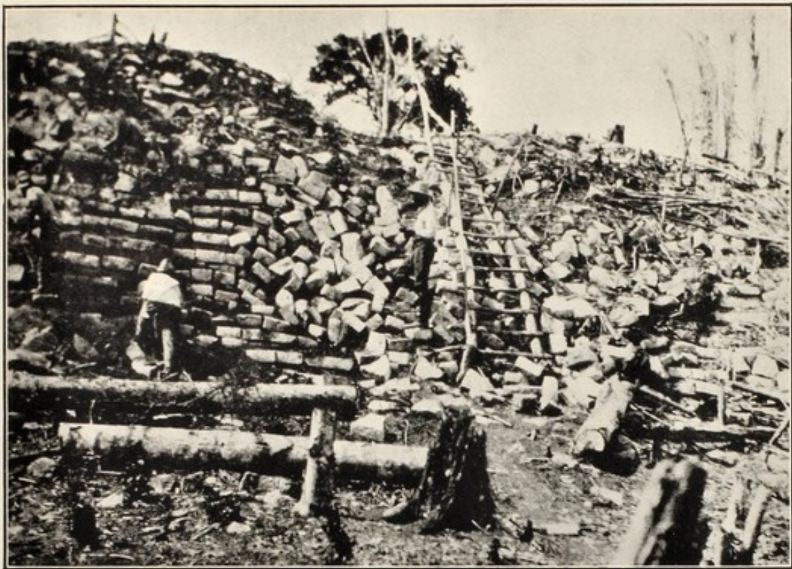
RUINED STAIRWAY AND BUSH LADDER
