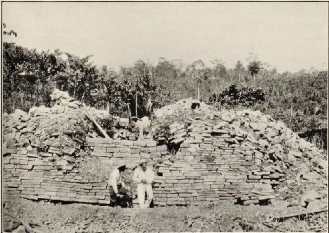
STONE-FACED PYRAMID SHOWING CORE AND OUTER SKIN
