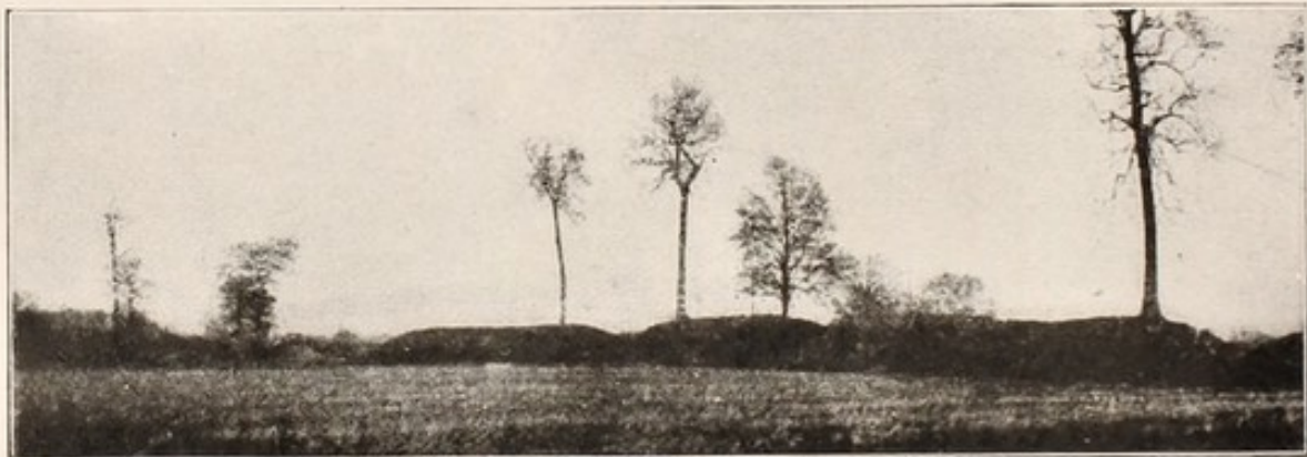
Section of East Wall, North Fort.
