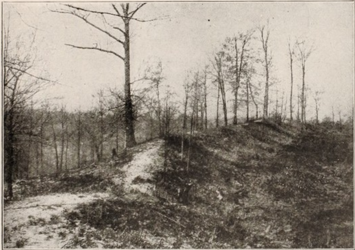
Section of South Wall, Old Fort.
