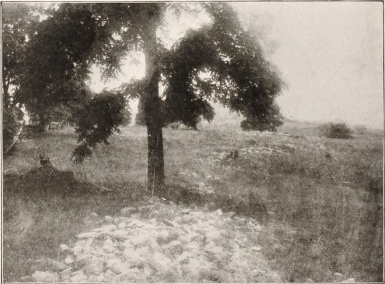
Glenford Fort — East Wall.
