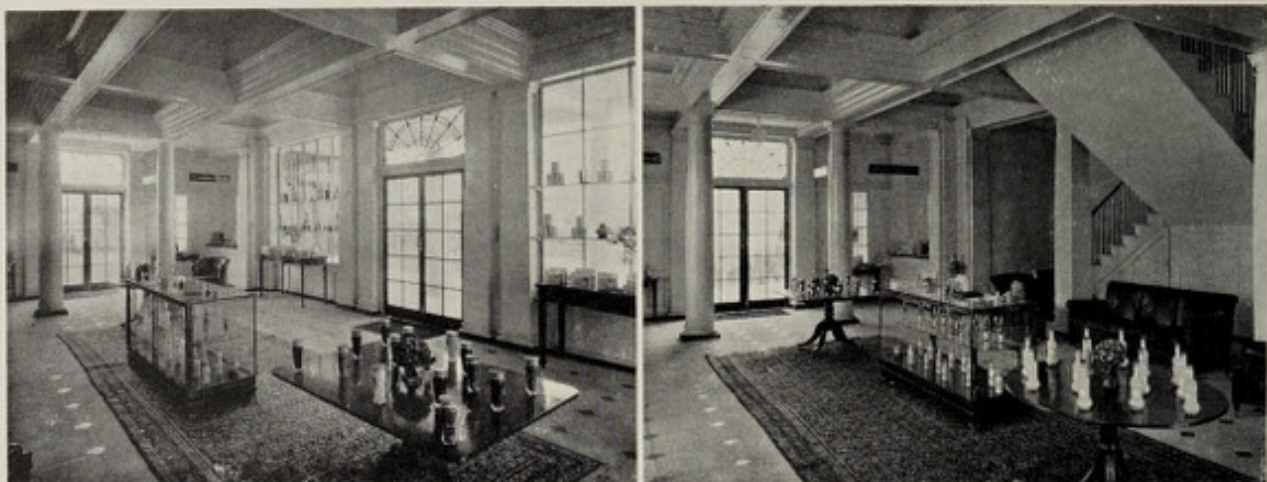
FIGS. 184 AND 185.—TWO VIEWS OF INTERIOR (GROUND FLOOR) CROSSE AND BLACKWELL'S PAVILION.
