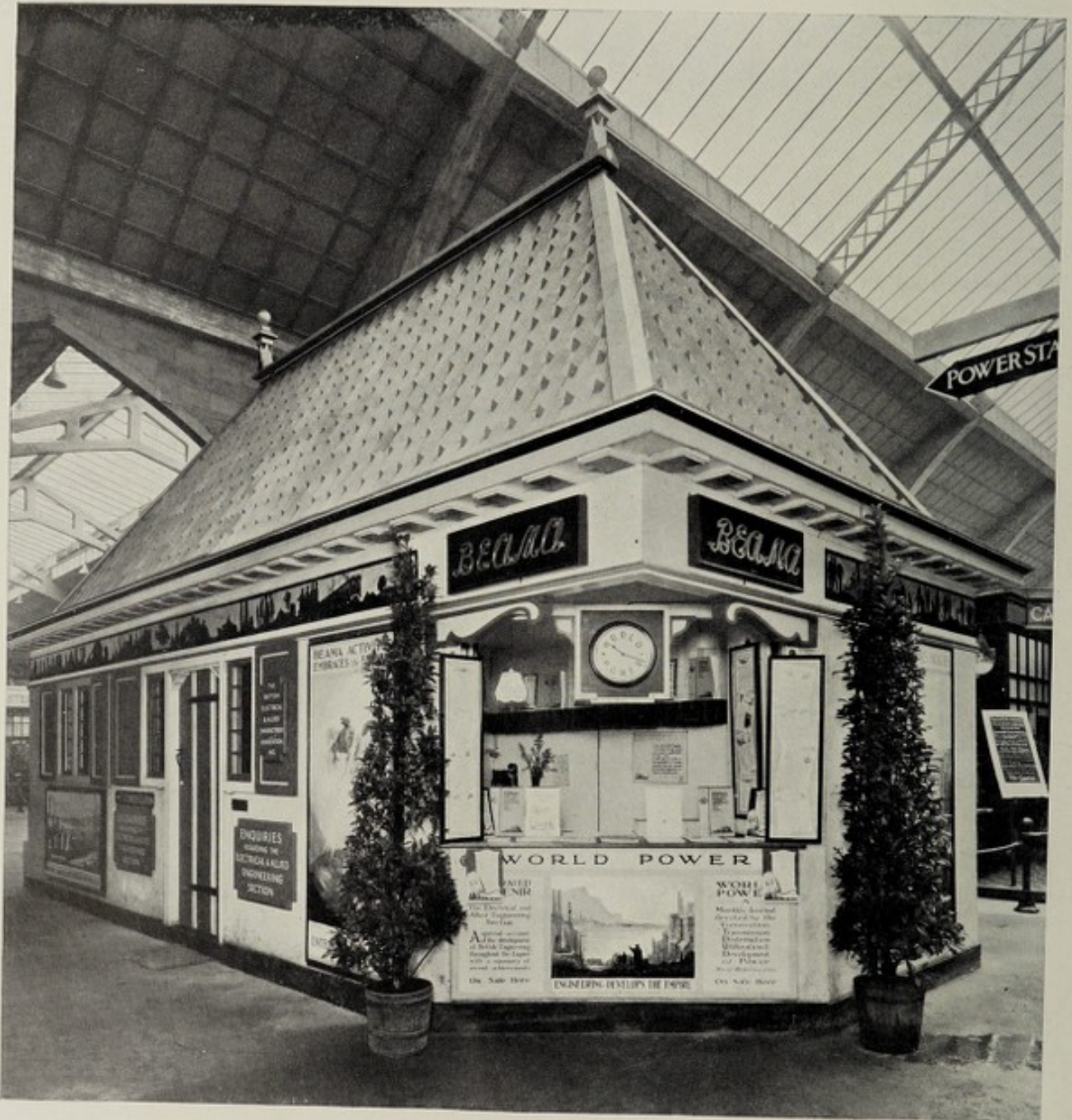
FIG. 254.—BEAMA OFFICE, PALACE OF ENGINEERING, WEMBLEY, 1924.
