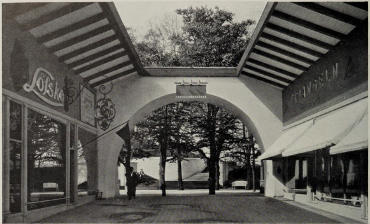
FIG. 8.—SHOPS ON BRIDGE OVER ROAD, GOTHENBURG EXHIBITION, 1923.
