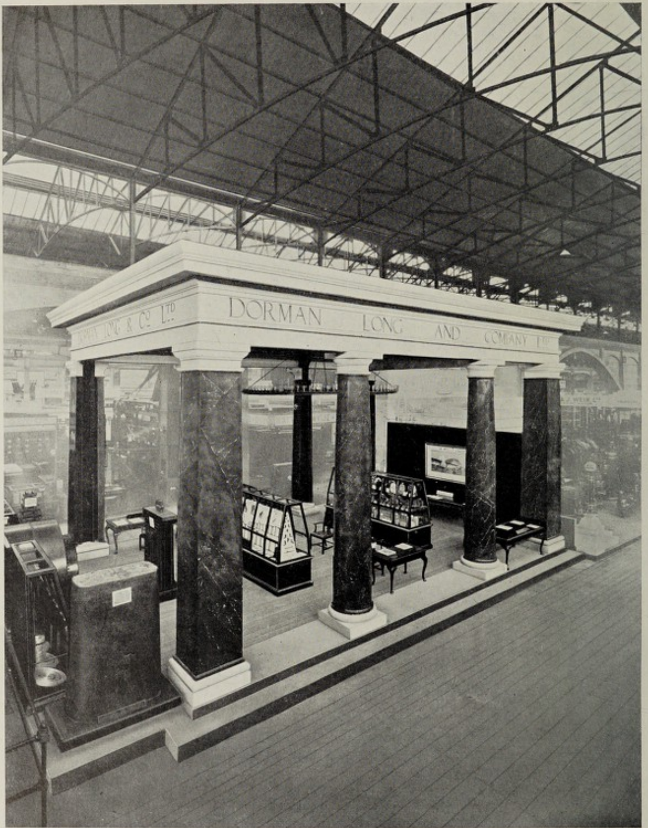
FIG. 144.—DORMAN LONG'S STAND, PALACE OF ENGINEERING, WEMBLEY, 1924: STEEL STANCHIONS INSIDE MARBLE COLUMNS.
