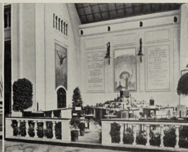
FIG. 65.—SMOKE ABATEMENT WEMBLEY.
