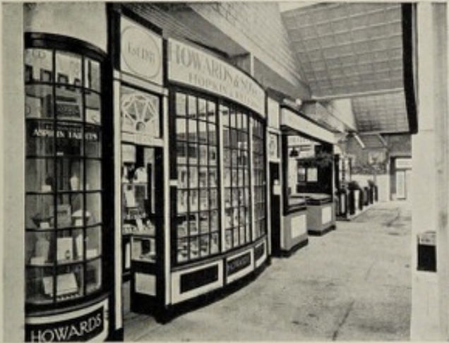
FIG. 230.—HOWARD'S OLD SHOP FRONT TREATMENT.
