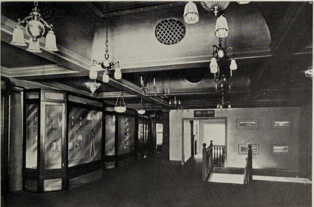
FIG. 273.—ON UPPER FLOOR OF G.E.C. PAVILION.
