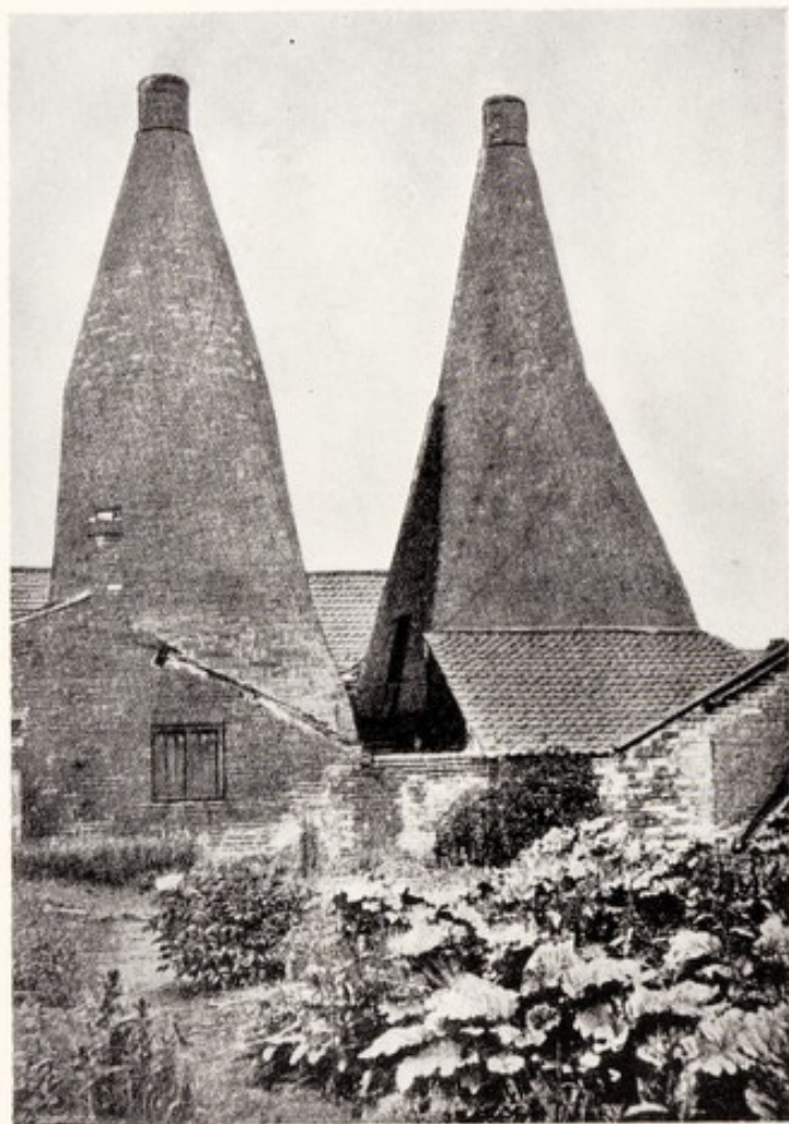
CEMENTATION FURNACES BUILT BY BENJAMIN HUNTSMAN ABOUT 1750.
