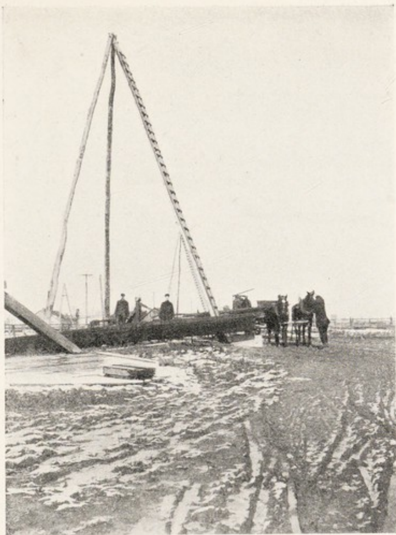
FIG. 77.—PETROLIA, CANADA. THREE-POLE DERRICK USED FOR CLEANING AND REPAIRING PUMPING WELLS.
