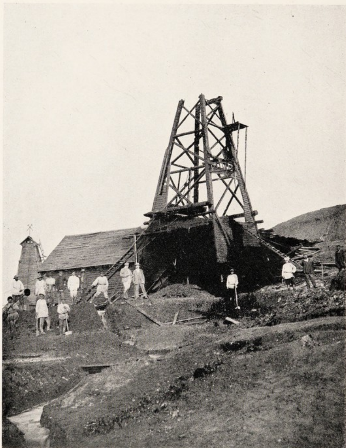
FIG. 92.—GROSNIC (S. RUSSIA) DERRICK AFTER DESTRUCTION BY OIL FOUNTAIN. AKHWERDOFF. No. 7.
