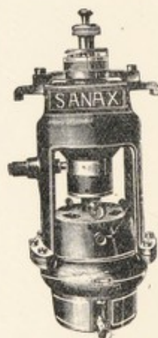
FIG. 17. Sanax interrupter.
