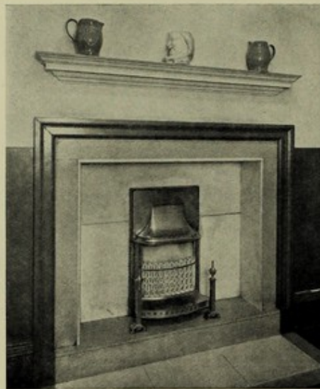
Fig. 10. Fire set 10\frac{1}{2} ins. behind front face of architrave which projects 2 ins. from the wall, giving a net recess of 8\frac{1}{2} ins.
