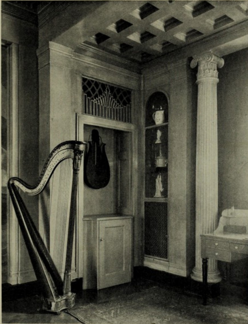
Fig. 38. Gas Radiator behind grille (below china cupboard) Architect: P. Morley Horder
