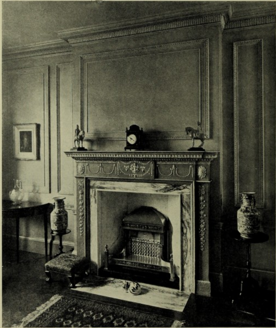
Fig. 19. At 39 Holland Street, Kensington. The drawing-room. Gas fire with canopy and dogs. Architect: H. Austen Hall, F.R.I.B.A.
