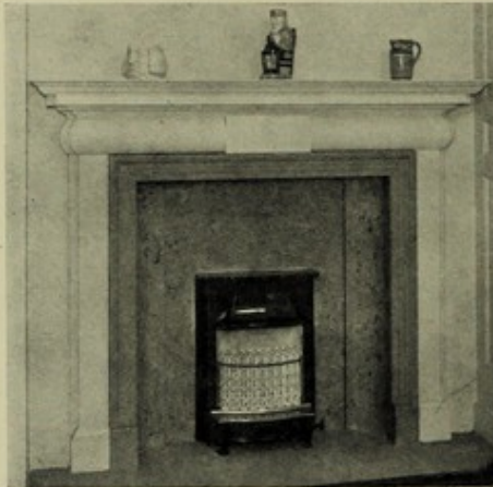
Fig. 9. Fire set 9\frac{1}{2} ins. behind front face of the marble surround which projects 4 in. from the wall, giving a net recess of 5\frac{1}{2} ins.
