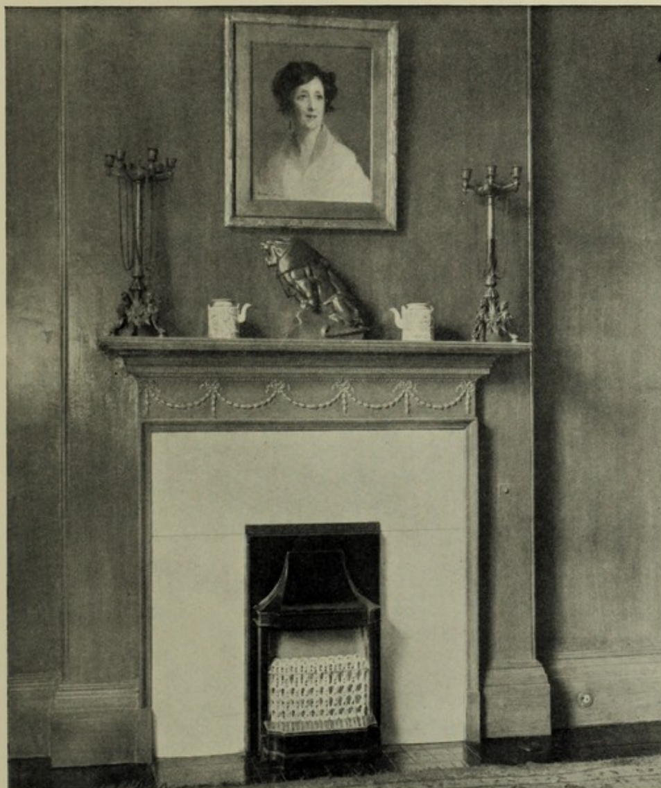
Fig. 35. A self-contained gas fire placed in front of a coal grate over which it fits exactly, involving no disturbance of existing surround. Architect: P. Morley Horder
