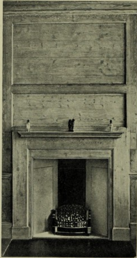
Fig. 31. At 9 Hanover Square, London, W. In a private office. Sloping type without interior frame Architect: Oliver Hill, F.R.I.B.A.
