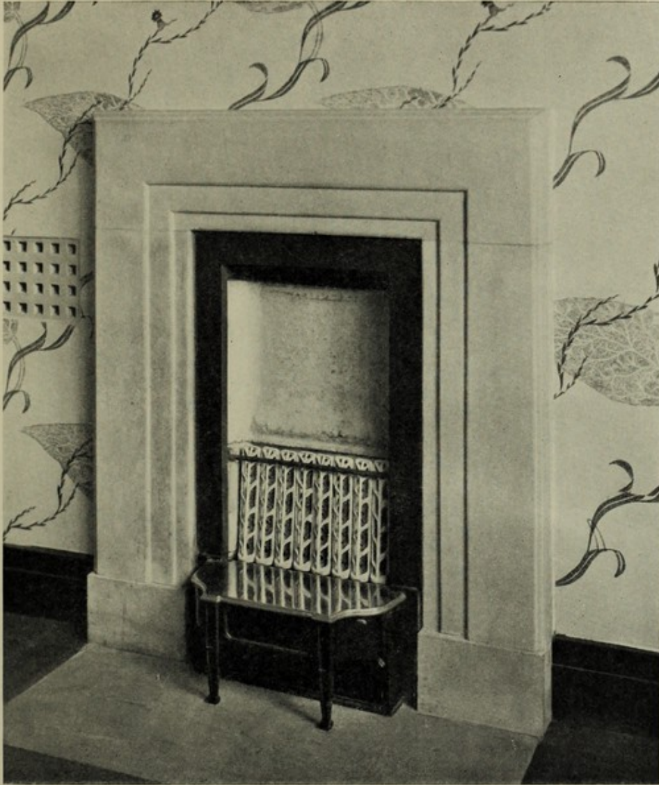
Fig. 14. At Mansard House, Loughton, Essex. Gas fire set in Hopton Wood Stone Architect: Edward Maufe, M.A., F.R.I.B.A.
