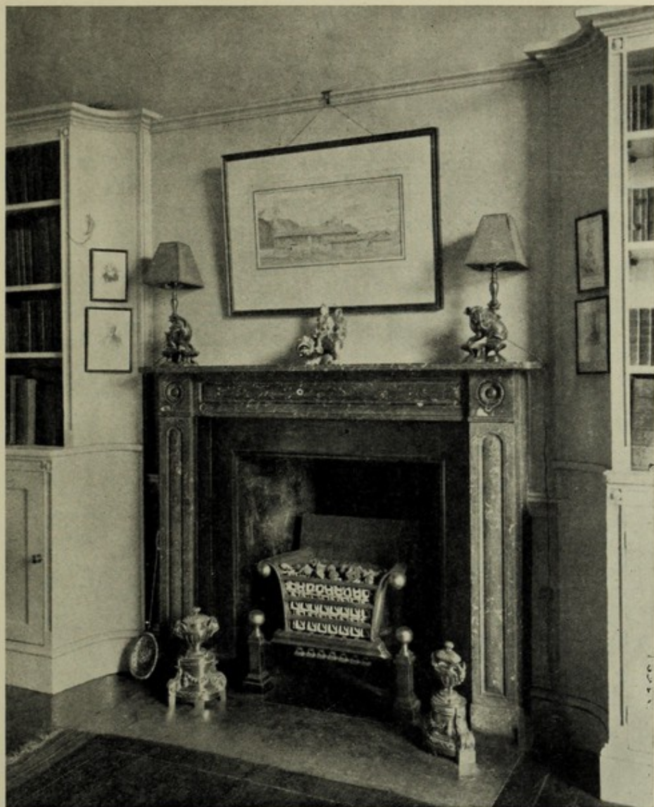
Fig. 36. Bedford House, Chiswick. The Study. A dog basket grate adapted to gas Architect: Darcy Braddell, F.R.I.B.A.
