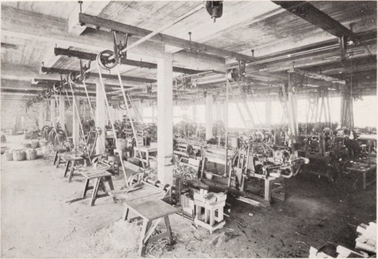
SARDINE CAN-MAKING PLANT.
