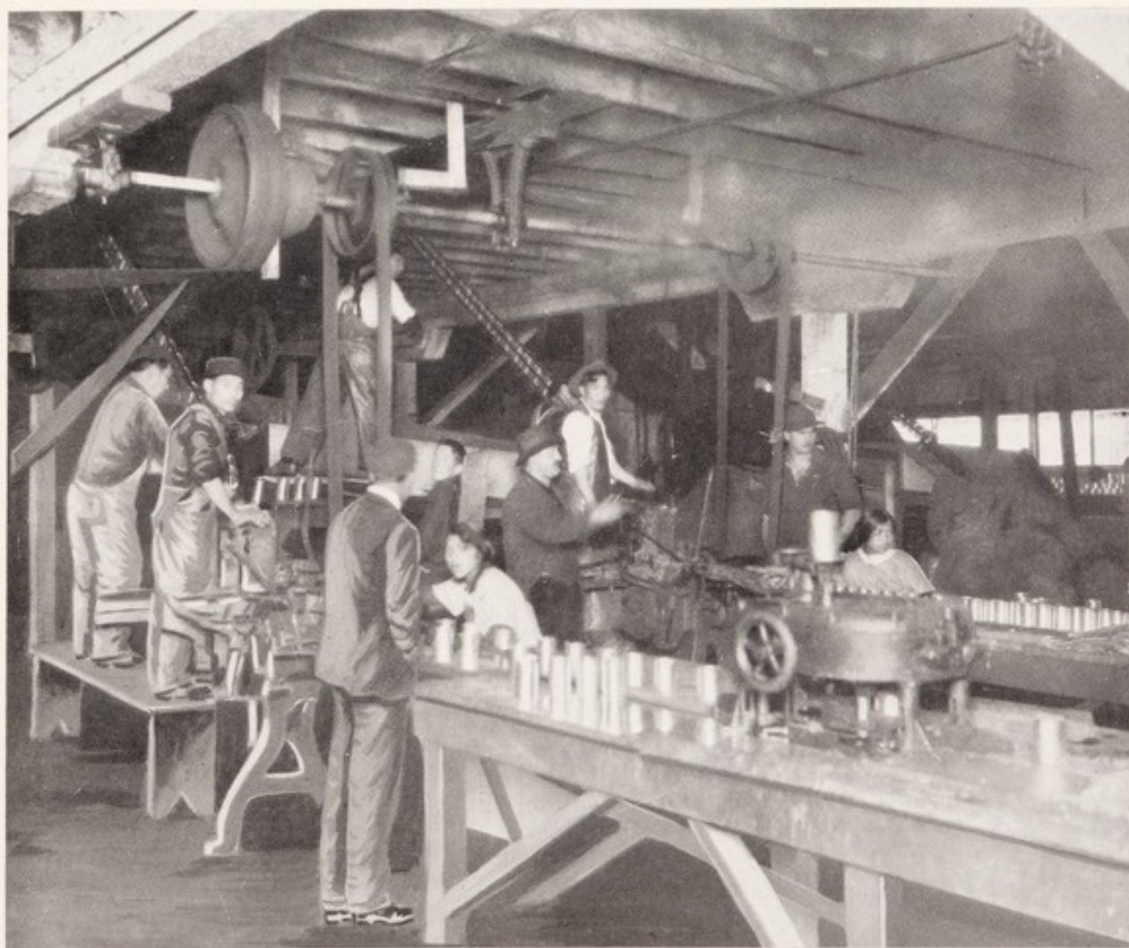
THE SALMON FILLING AND WEIGHING MACHINES.
