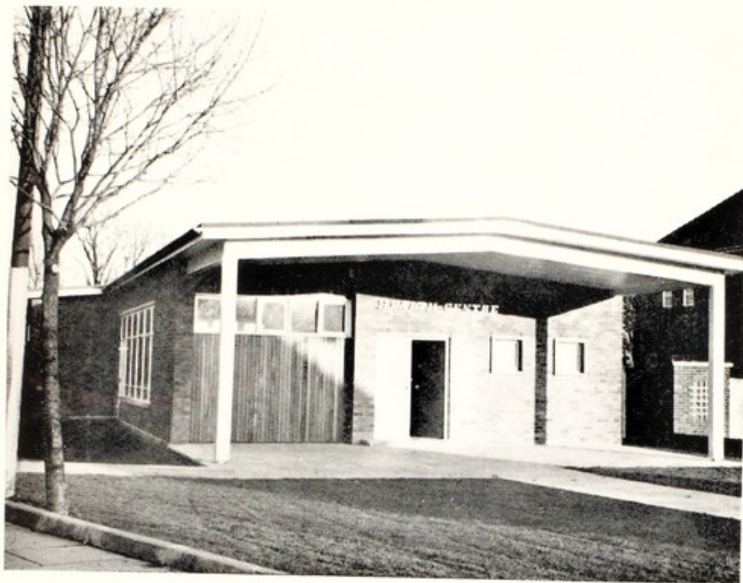
2. Entrance to Gooseberry Hill Centre
