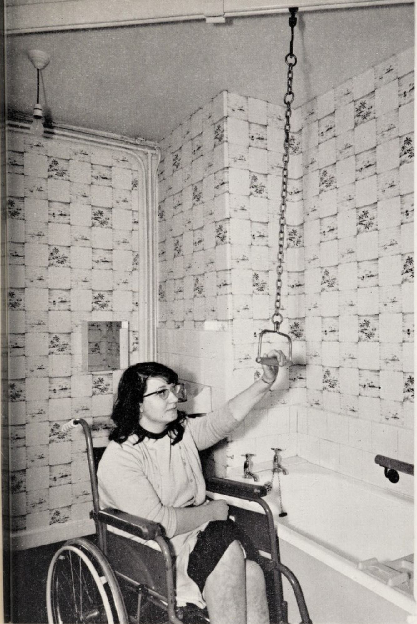
bi/Aids for Handicapped. girl This special bathroom was constructed by dividing part of for the kitchen in a local authority dwelling. A low bath, handrails and lifting apparatus have made this patient completely independent
