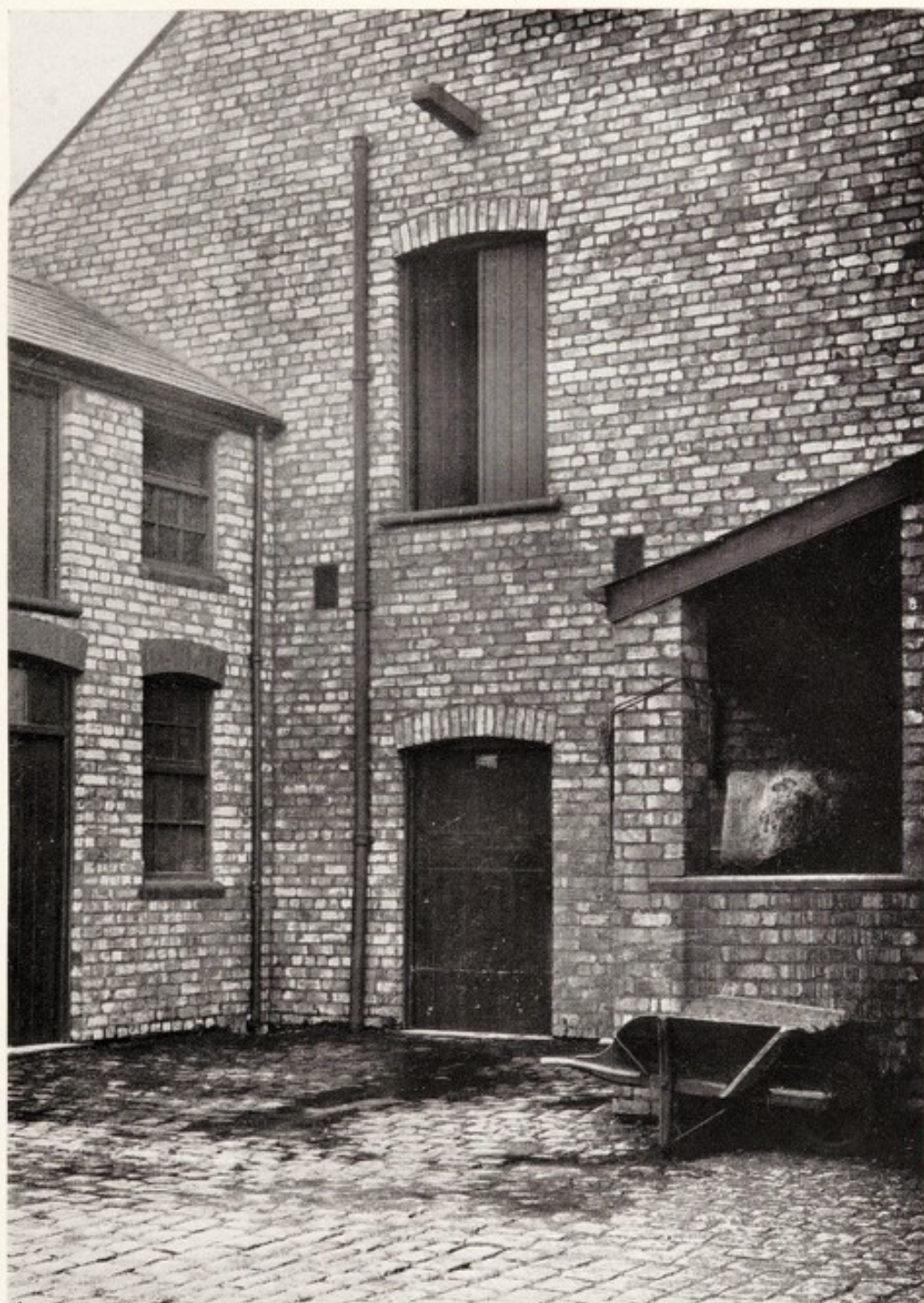
EXTERIOR VIEW OF A TOWN COWSHED SHOWING MIDDENSTEAD.
