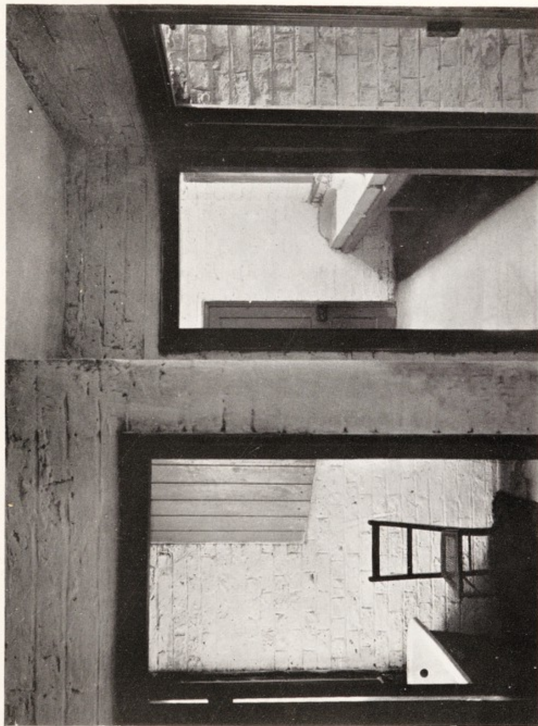
COMMON LODGING HOUSE FOR WOMEN, EVERTON BROW. Lavatory and Bath Accommodation.
