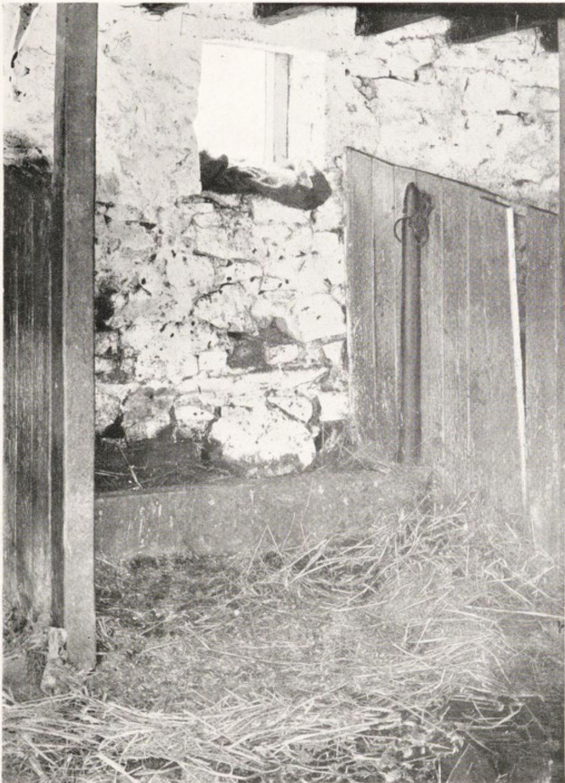
A Denbighshire Cowshed from which Tubercular Milk was sent into Liverpool, the premises being deficient in light, ventilation and cleanliness. Practically the only light and ventilation is from the doors, and when these are closed the place is without light or ventilation. An order was made prohibiting the supply of Milk from this Cowshed to the City of Liverpool.
