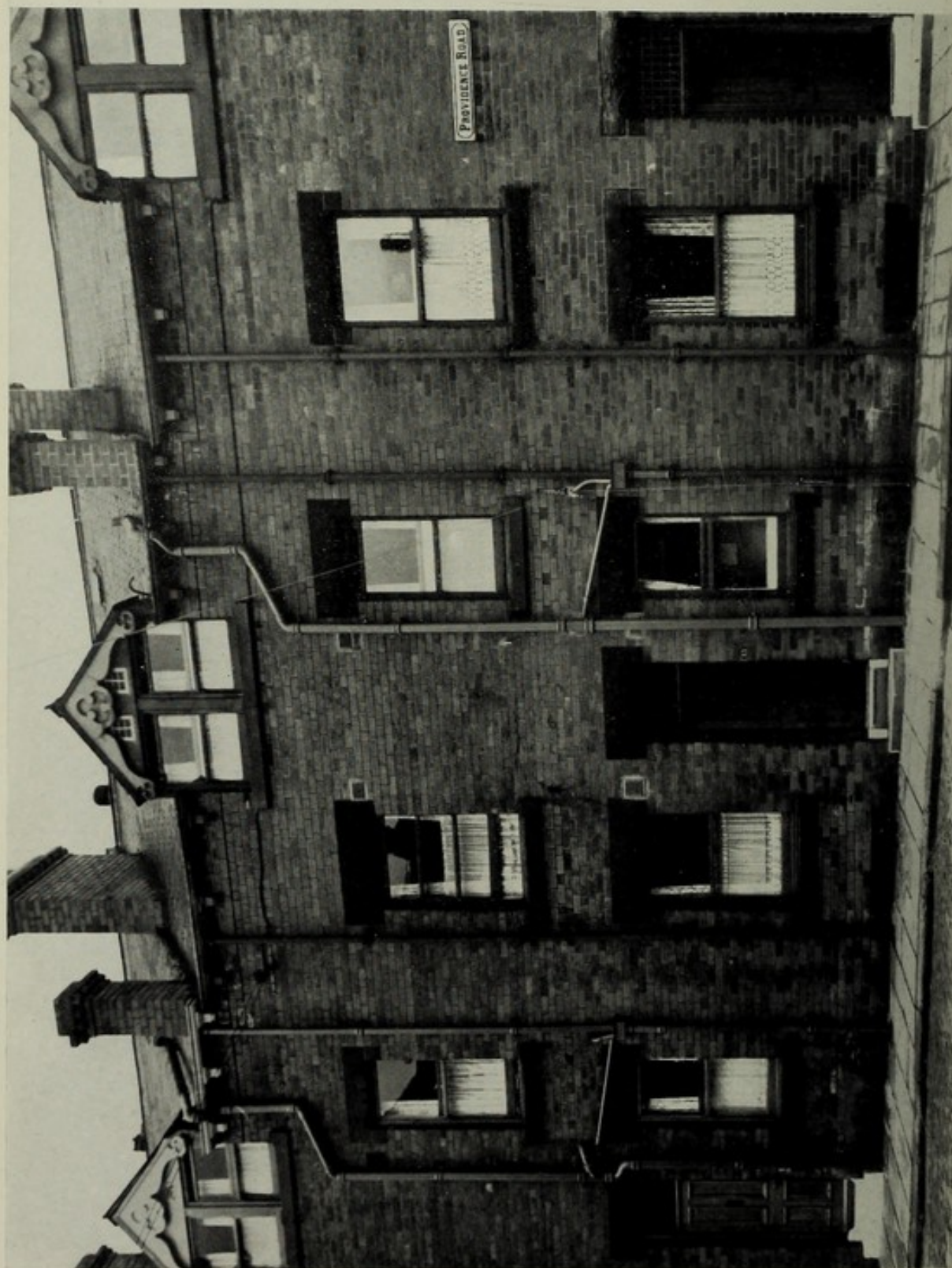
Photograph, after improvement, of external elevation showing air inlets of No. 13, Providence Road, Leeds, 6.
