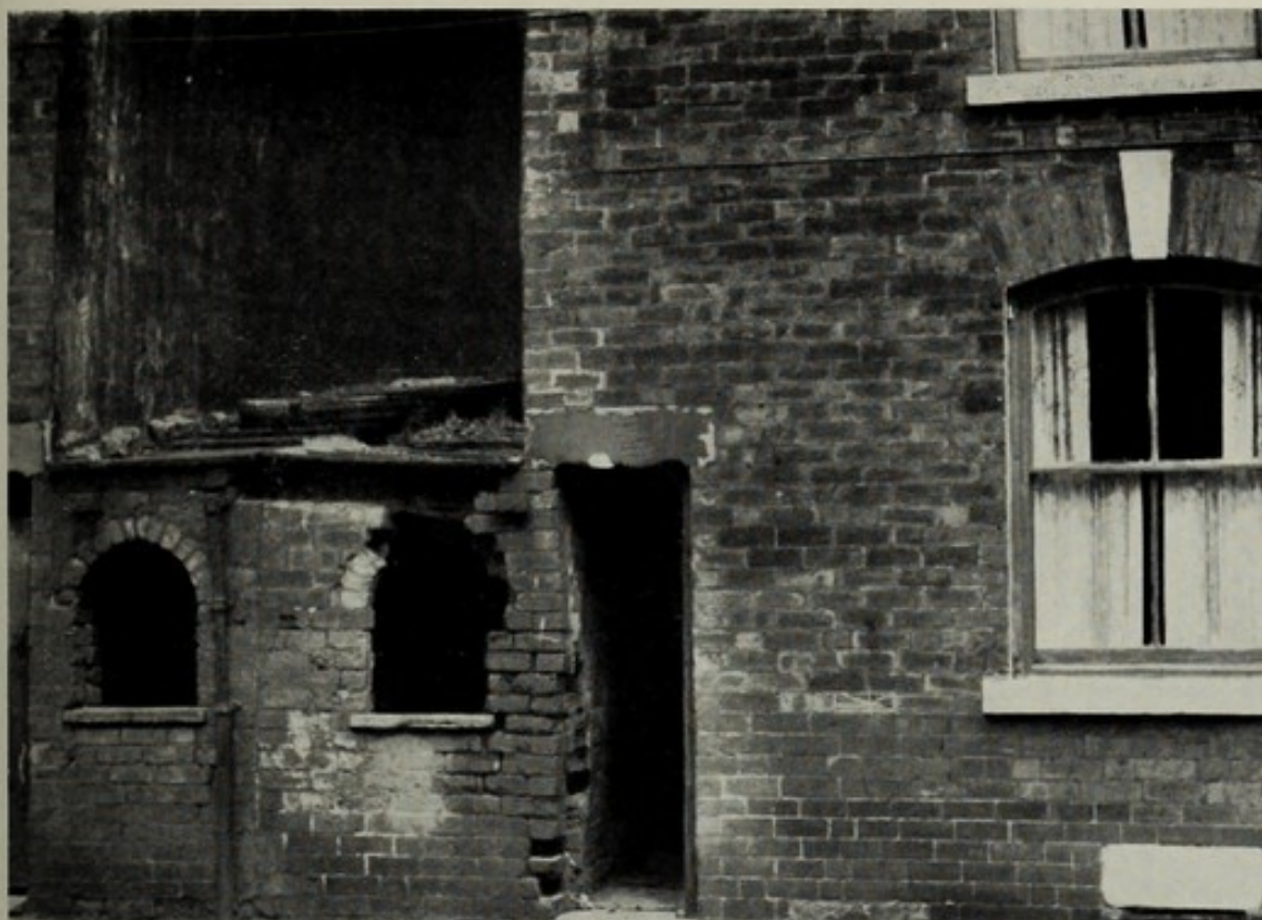
These two ashpits served eight houses. The structures were dangerous, the roofs leaked and the wetted foul contents escaped through broken brickwork to foul the footways. Ashpits abolished as shown below.
