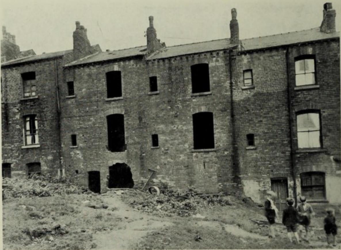
REAR OF 12, GLOVER STREET. Derelict house being used as a dumping ground for offensive refuse. Demolition Order made October, 1951.
