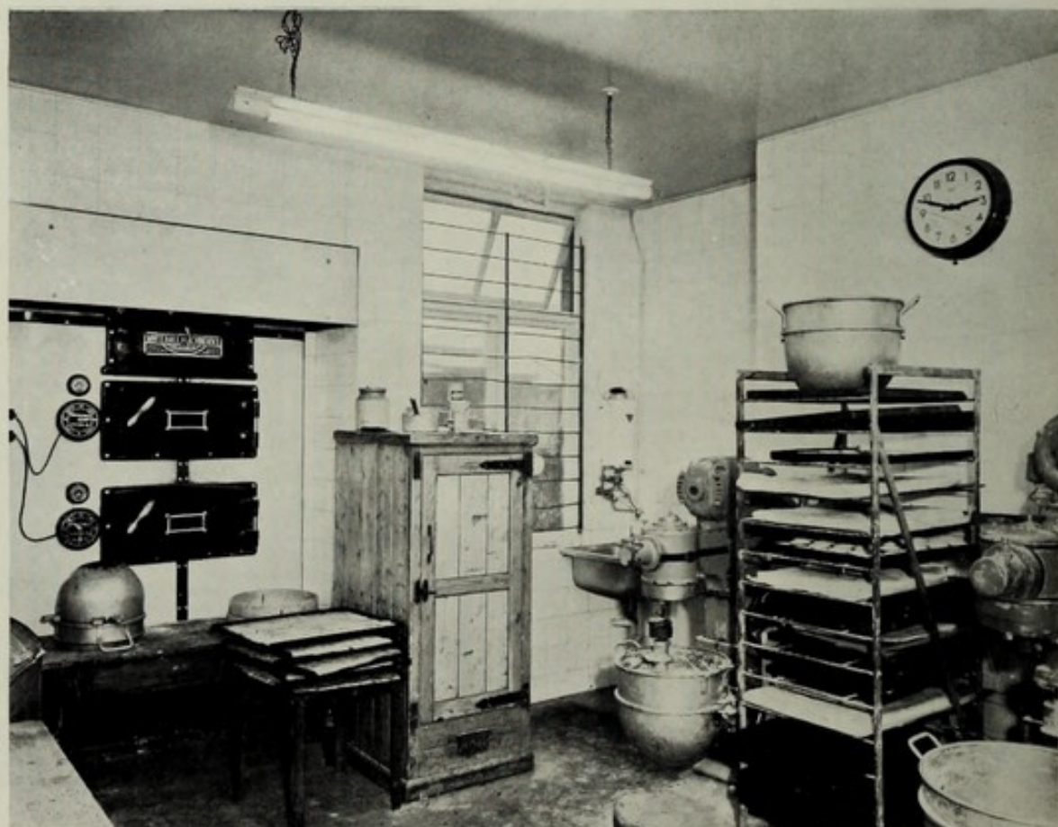
New bakehouse constructed in ground floor to replace bakehouse shown in top photograph. Showing composition floor, tiled walls, painted ceiling, adequate natural lighting and ventilation, stainless steel sink with constant supply of hot and cold water, mechanical extraction for steam from oven.
