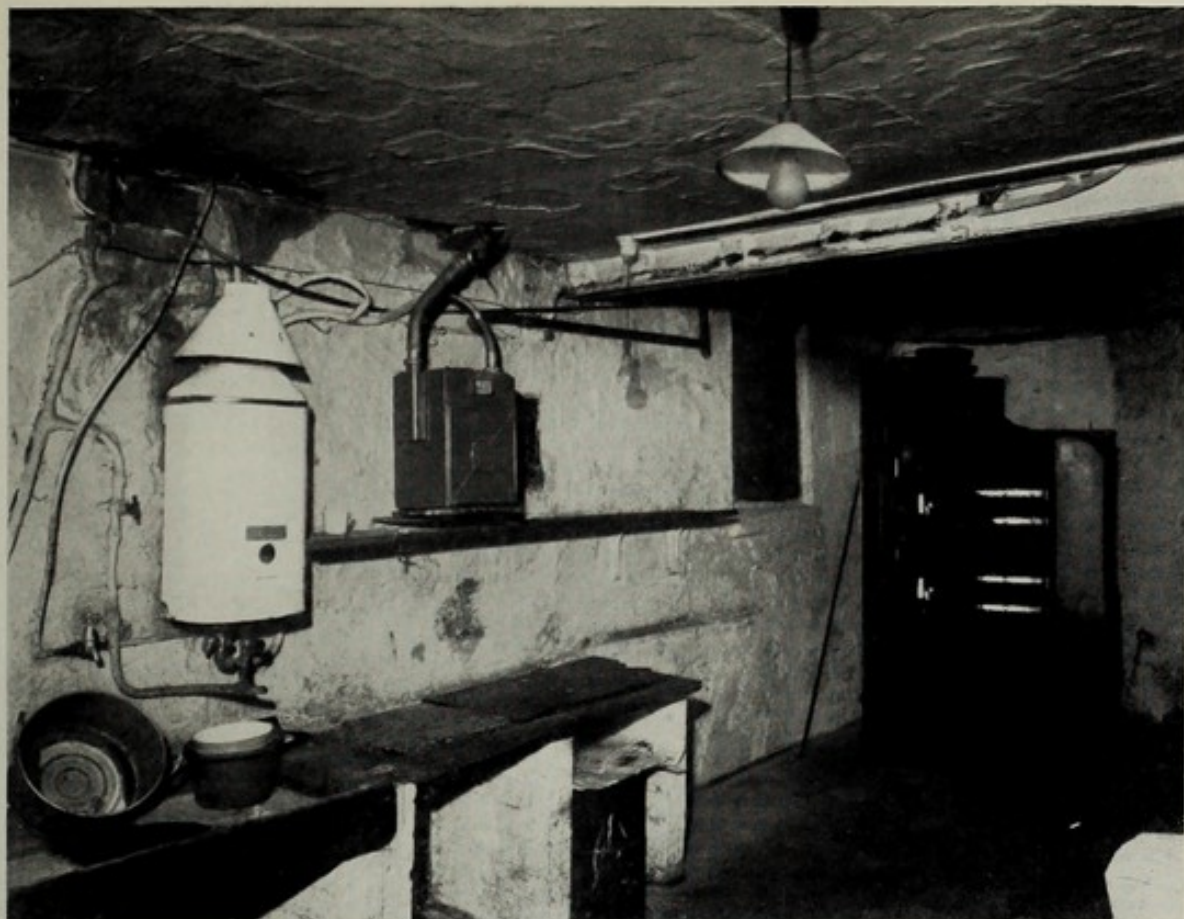
Basement bakehouse, entirely below ground level, showing unsatisfactory state of walls and ceiling, inadequate natural lighting and ventilation and unglazed sink. Bakehouse now disused. Photograph taken by flashlight.
