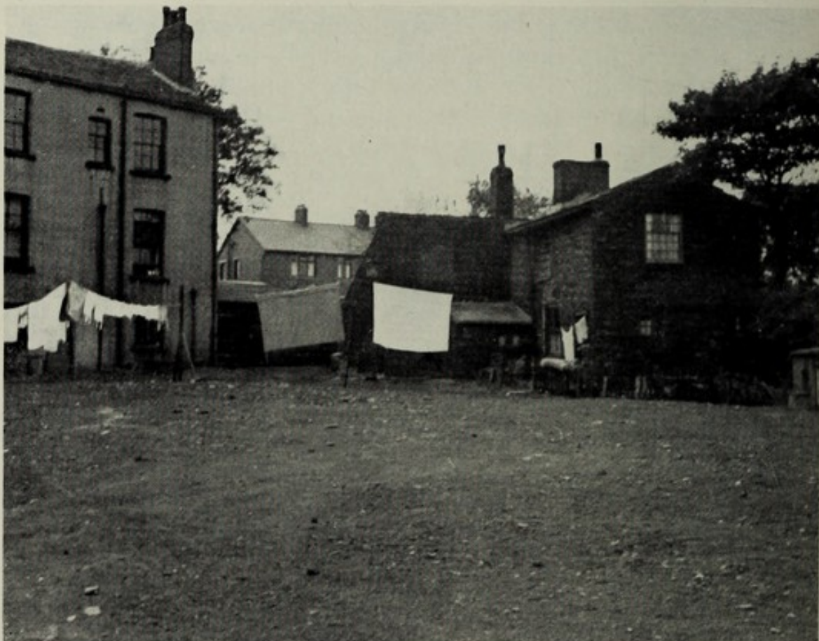
DEMOLITION OF INSANITARY HOUSES—HODGSON YARD. Cleared site of Nos. 3, 4, 5, 6, 7, 8, 9, Hodgson Yard. All cellars have been filled, drain openings sealed and site levelled and compacted.
