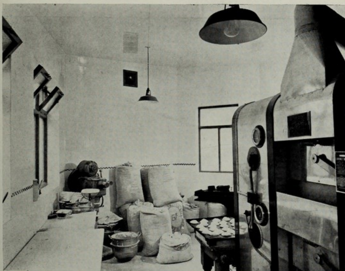
Above ground bakehouse newly built to replace basement bakehouse illustrated above, showing impervious floor, tiled walls, painted ceiling, good natural lighting with adequate ventilation and extract for steam from oven. Modern glazed sink (not shown) with constant supply of hot and cold water.
