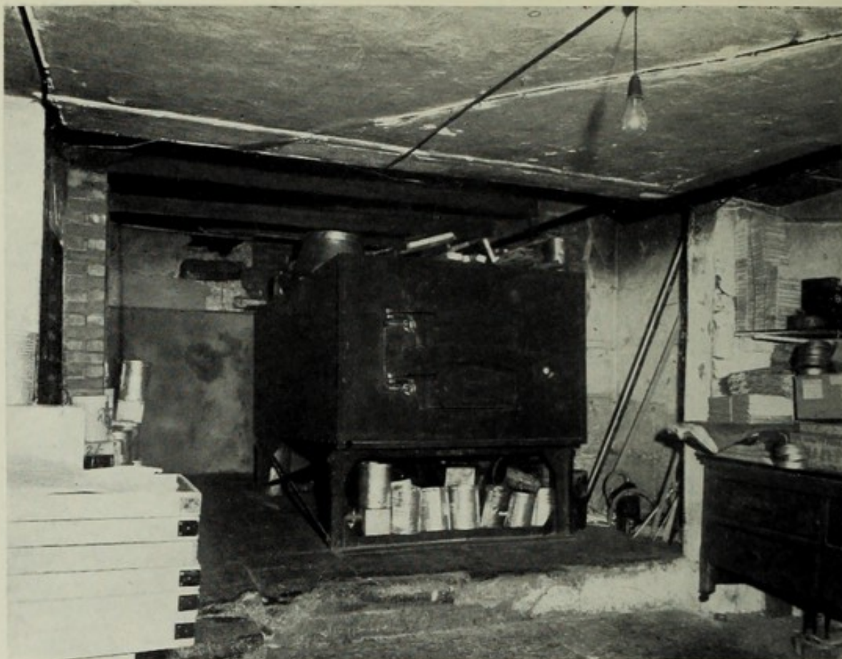
Basement bakehouse, showing defective floor, unsatisfactory condition of walls and ceiling, and inadequate lighting and ventilation. Bakehouse unprovided with a sink or with means of drainage at floor level, or with a constant supply of hot and cold water.
