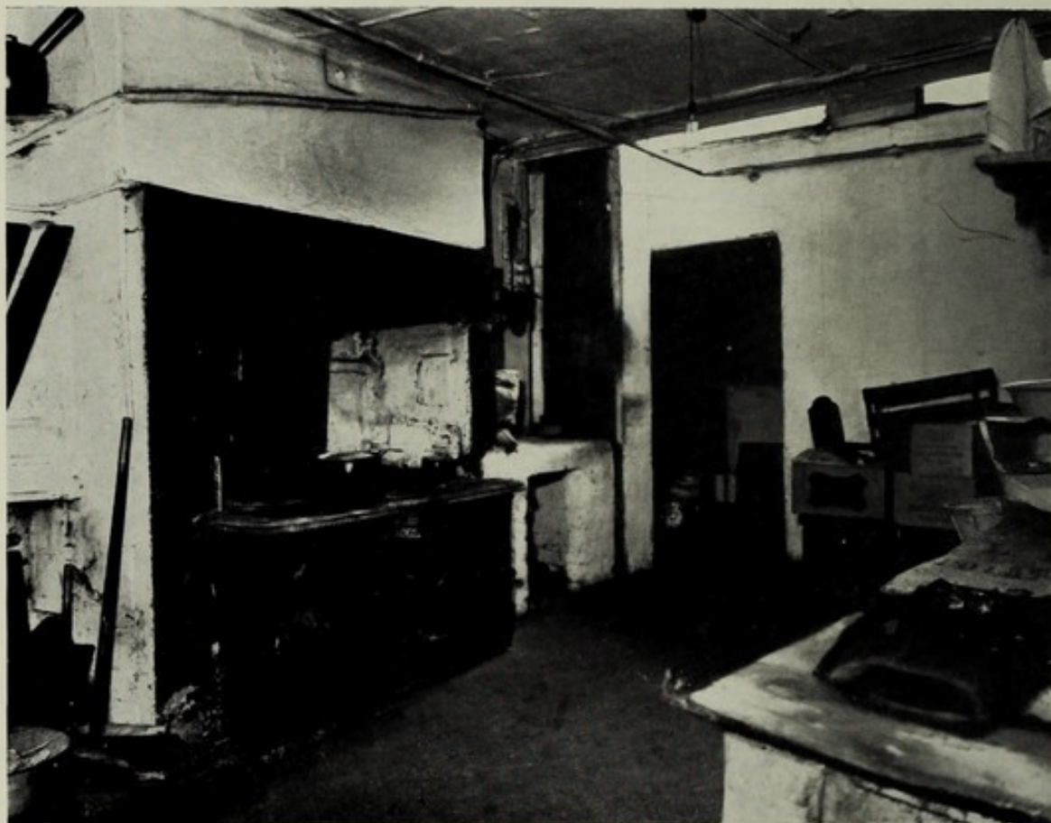
Dark underground kitchen, taken by flash-light, showing dilapidated stove, defective ceiling, worn floor, lack of natural light and ventilation, and general insanitary conditions.
