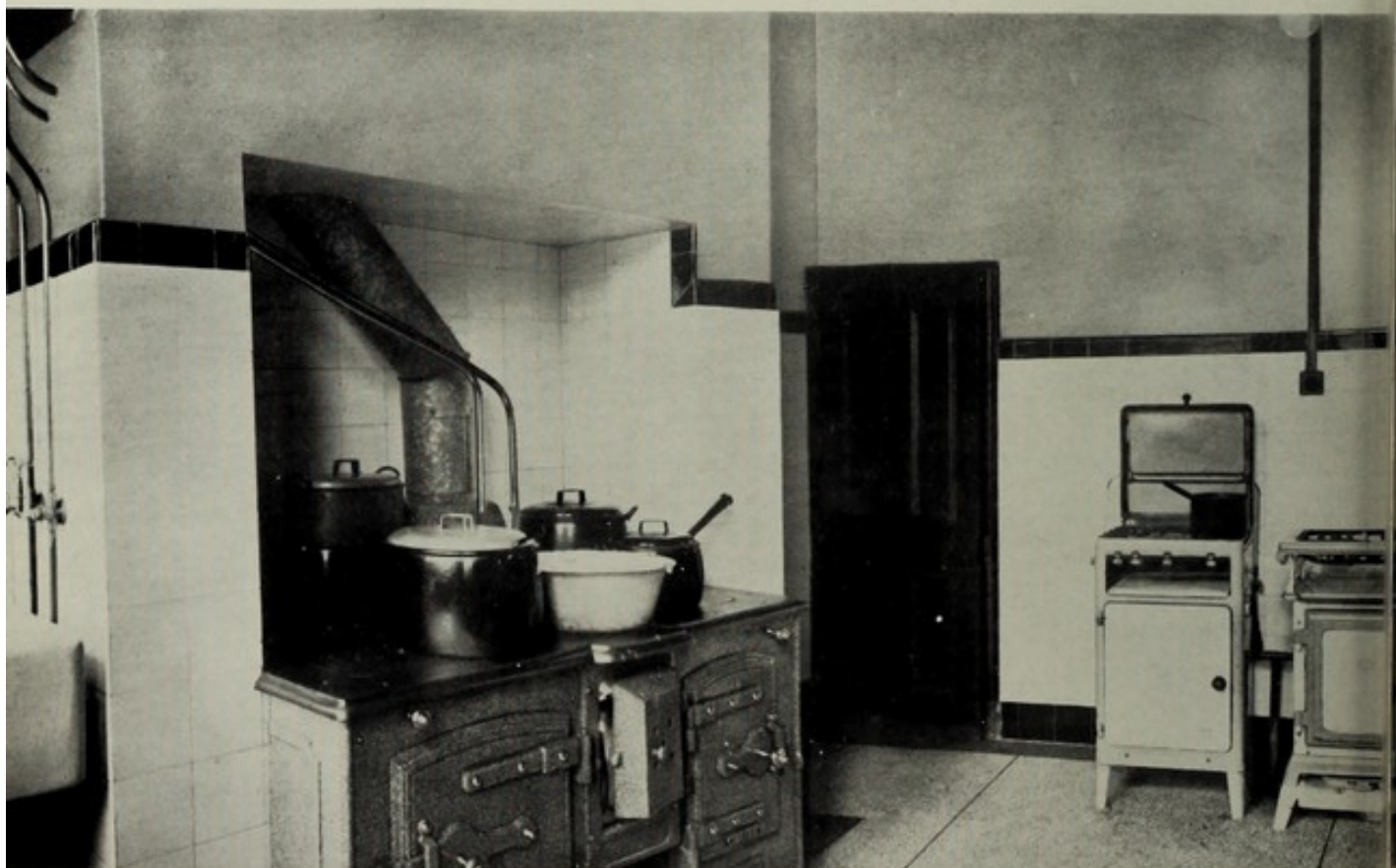
Kitchen transferred to Ground Floor. Room showing Tiled Walls, Terazzo Floor. New equipment and hot and cold water for the washing of hands.
