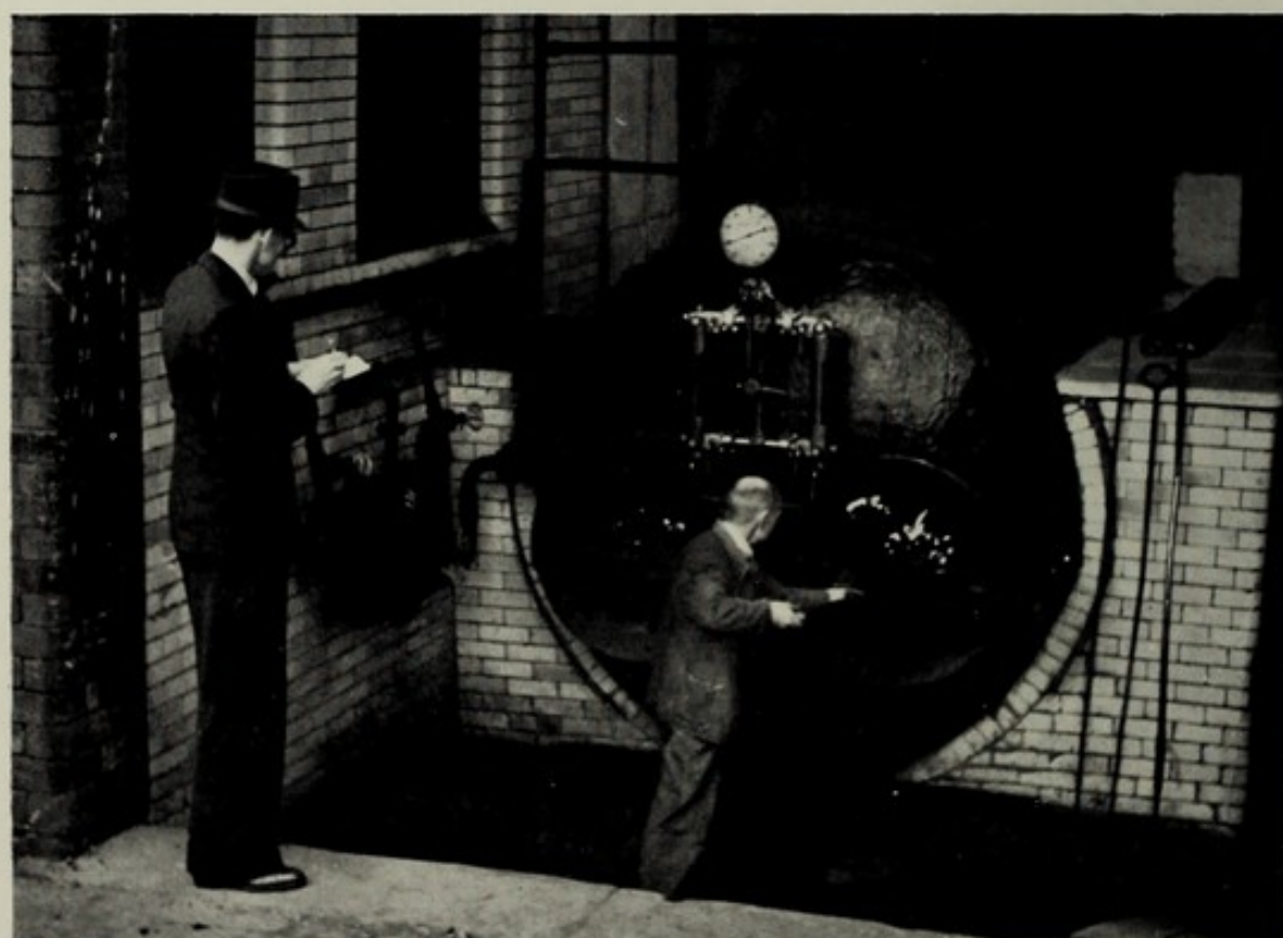
BOILER PLANT INSPECTION Inspector noting method of hand firing employed.
